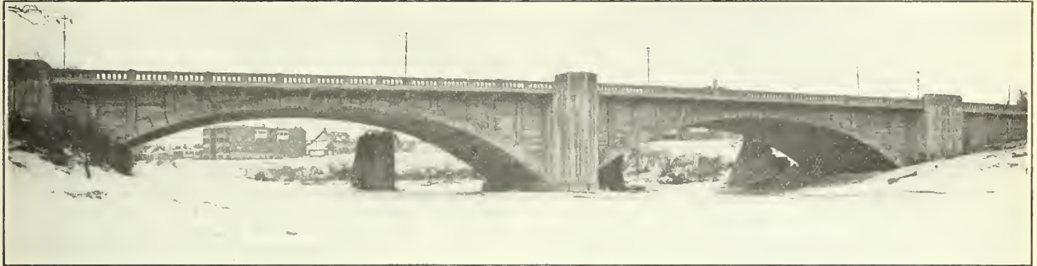
Fig. 5 Complete bridge with light poles erected and street cars operating over bridge.
