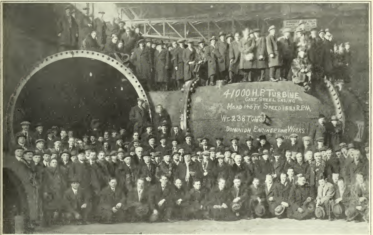
Members of The Engineering Institute of Canada photographed at the Dominion Engineering Works Limited at the time of the Annual Convention of the Institute, showing the metal turbine cast steel scroll casing for the forty-one thousand horse power turbine, the largest of its kind ever manufactured, having a weight of two hundred and thirty-eight tons.
