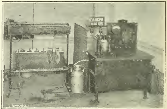
60,000 Volt Test Set for Testing Transformer Oil, Rubber Gloves, etc.
