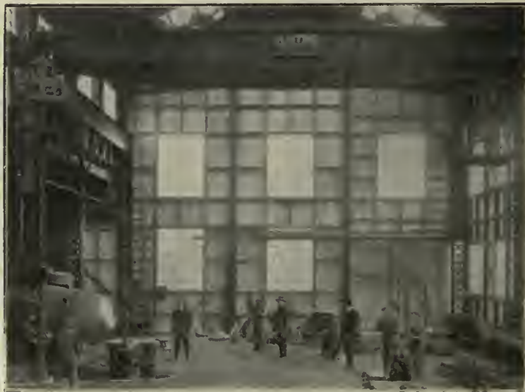
Fig. 4.—Ladle Lowered to Receive Finished Steel.
