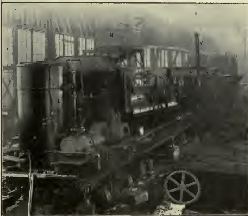
Cummer Portable Asphalt Plant
