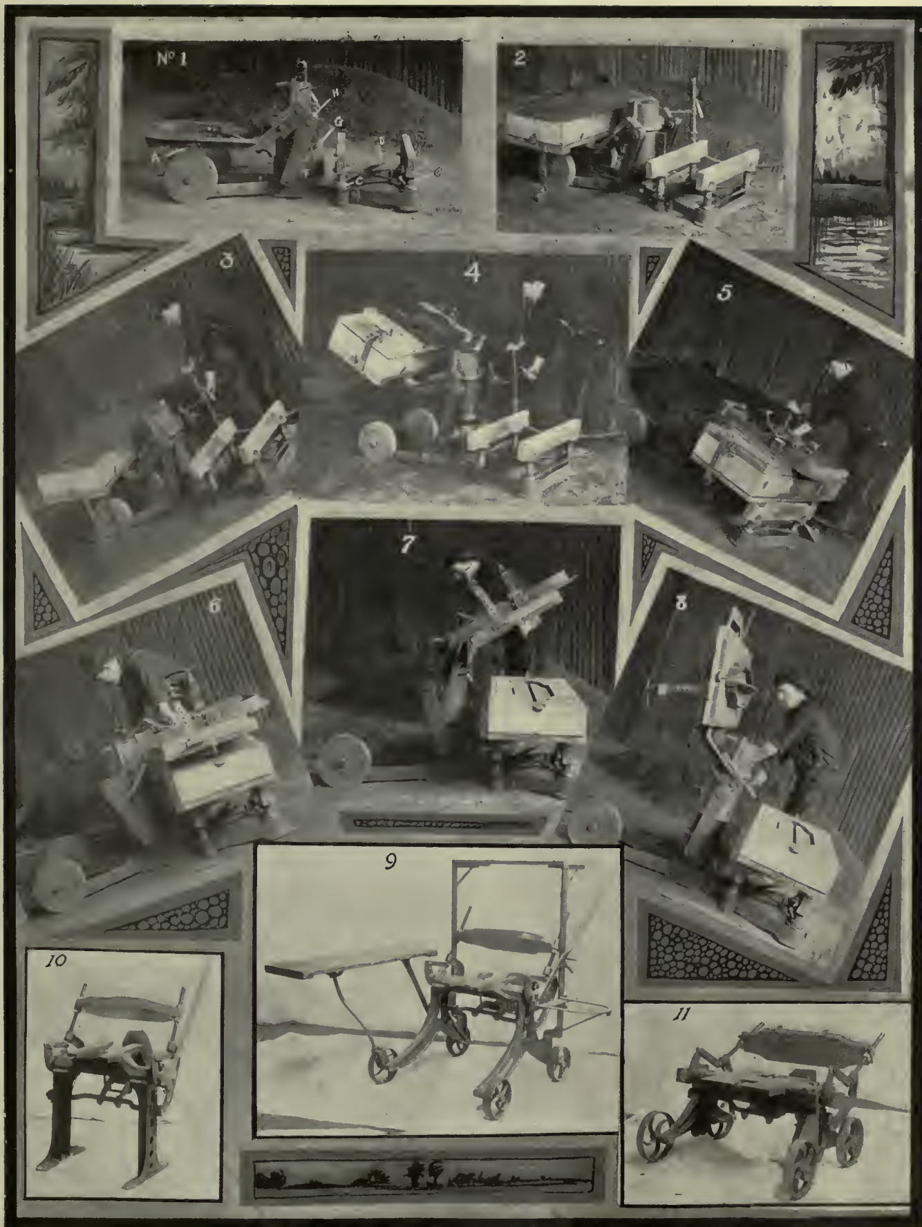
Fig. 1.—Farwell Pneumatic Roll-Over, Molding Machine. Fig. 2.—Flask in Place, Farwell Molding Machine. Fig. 3.—Operation of Jolting, Farwell Molding Machine. Fig. 4.—Raising Mold to Dead Centre, Farwell Molding Machine.
