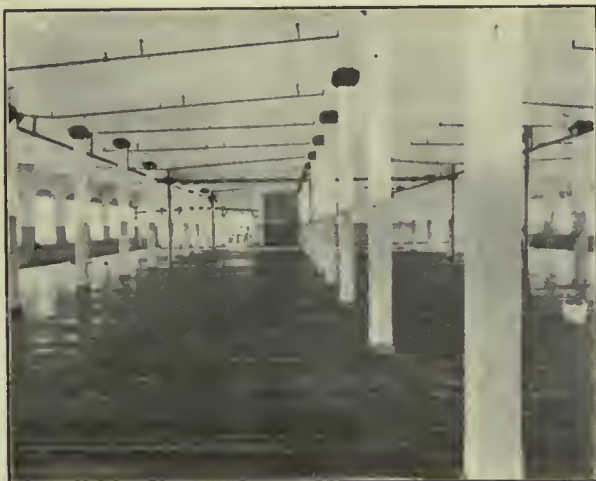
Construction of Fairbanks-Morse New Warehouse.
