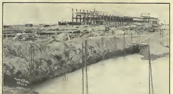
Fig. 4.—Steel Frame of Locomotive Shop.
