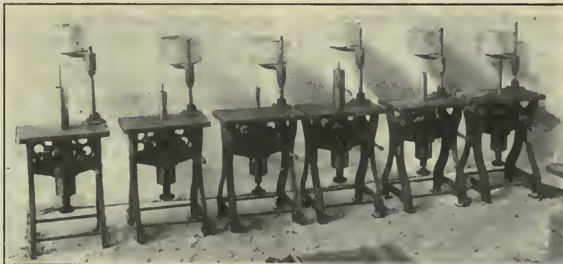
Fig. 5.—Machines Ready for Ramming Cores.
