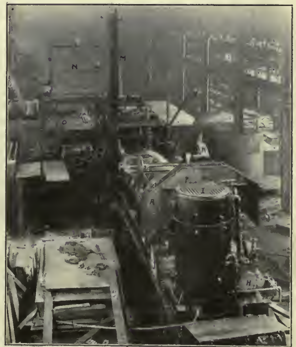
Cummer Portable Asphalt Plant
