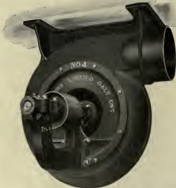
Fig. 3.—A Reversible Exhauster, Bolted to the Ceiling and Discharging Horizontally.
