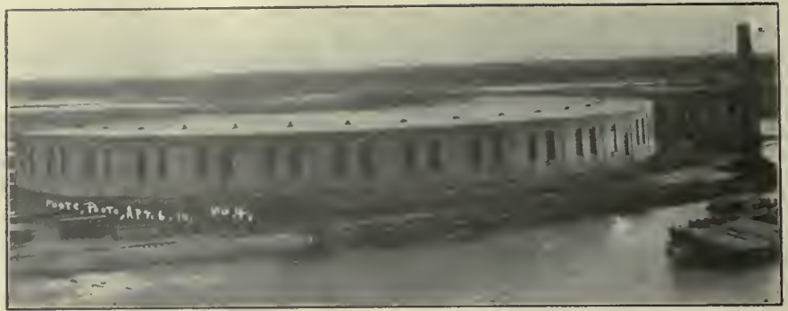
The Roundhouse in Connection with G.T.P. Shops.
