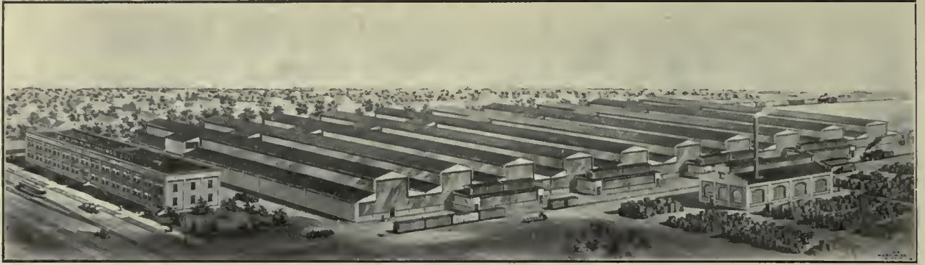
The Large Foundry of the Aluminum Castings Co., Detroit.
