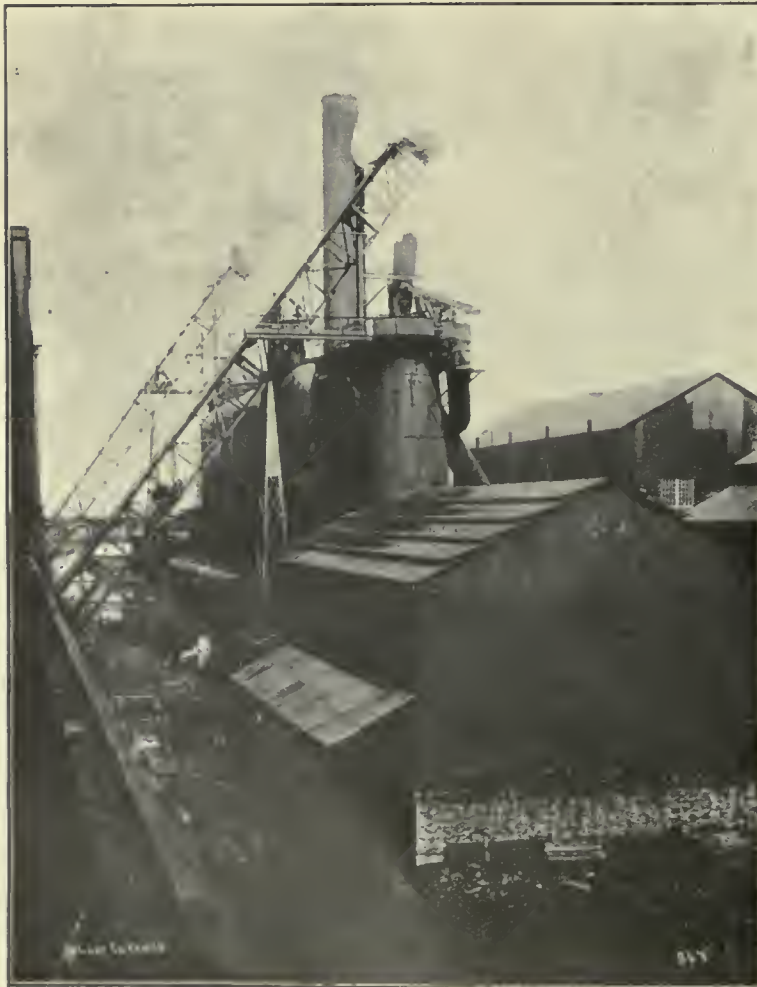
Blast Furnace Plant, Lake Superior Corporation, Sault Ste. Marie.
