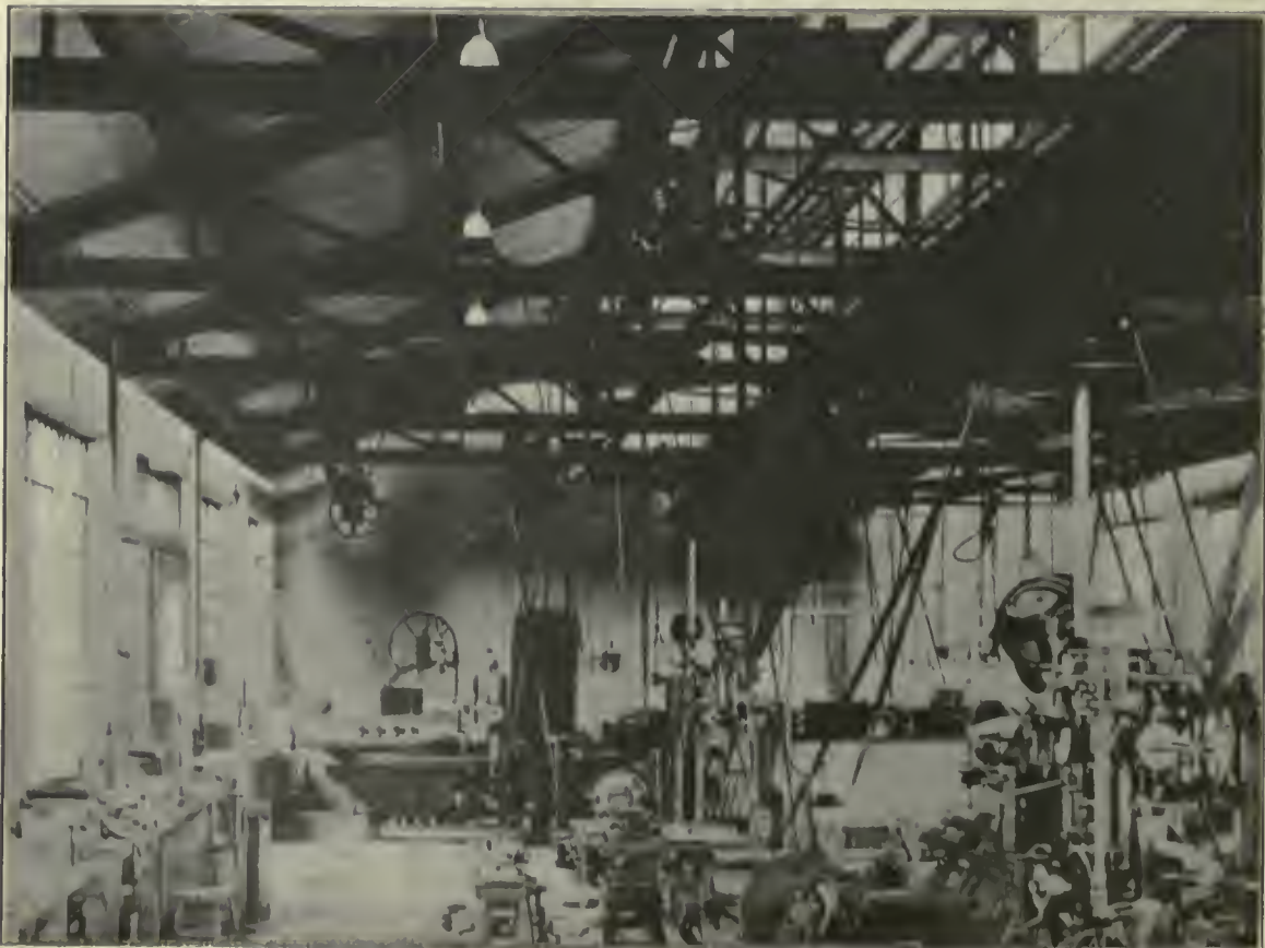
Fig. 2.—A Machine Shop, Showing General Illumination from 100-Watt Tungsten Lamps with Holophane Intensive Reflectors.
