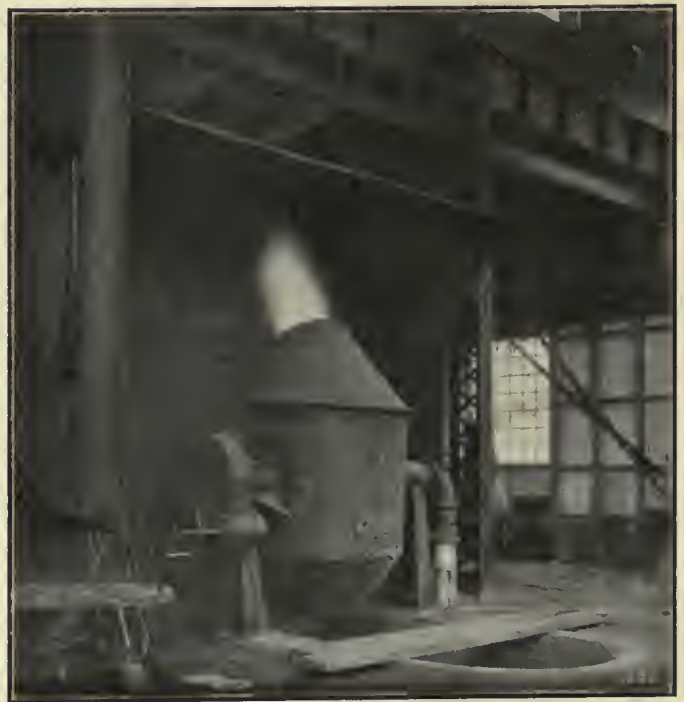
Fig. 5.—Converter During Progress of the Blow.
