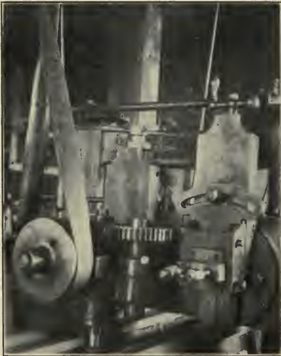
Fig. 1.—Milling Machine Milling on a Planer.
