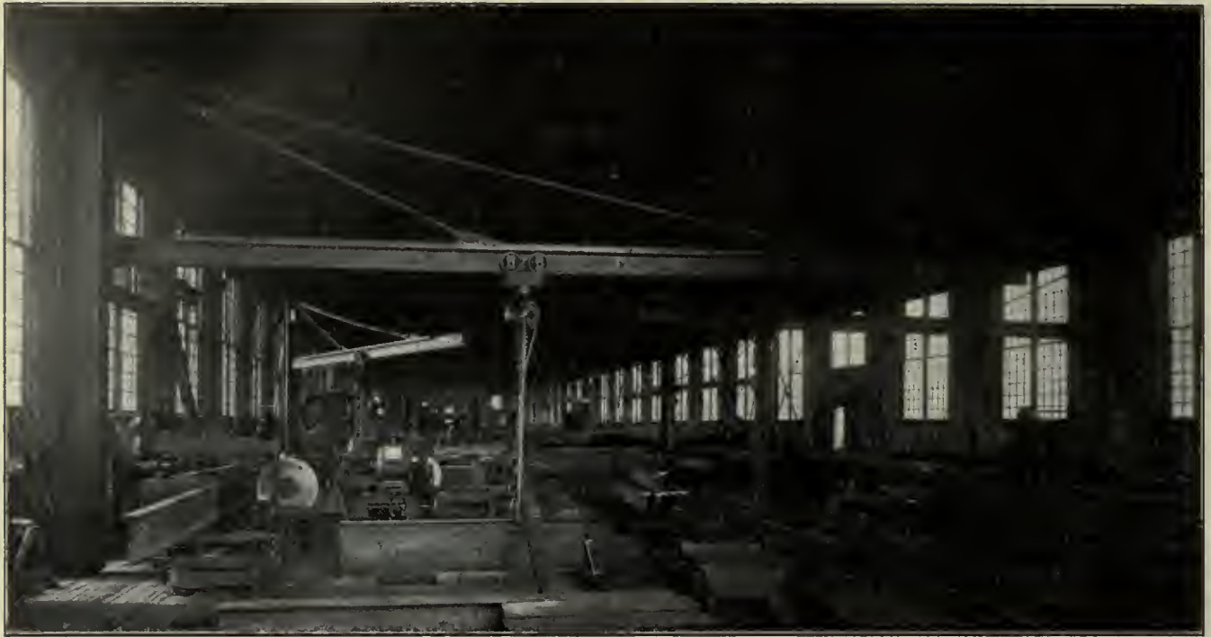
Interior Dominion Bridge Works, Toronto, Showing Facilities for Handling Material.
