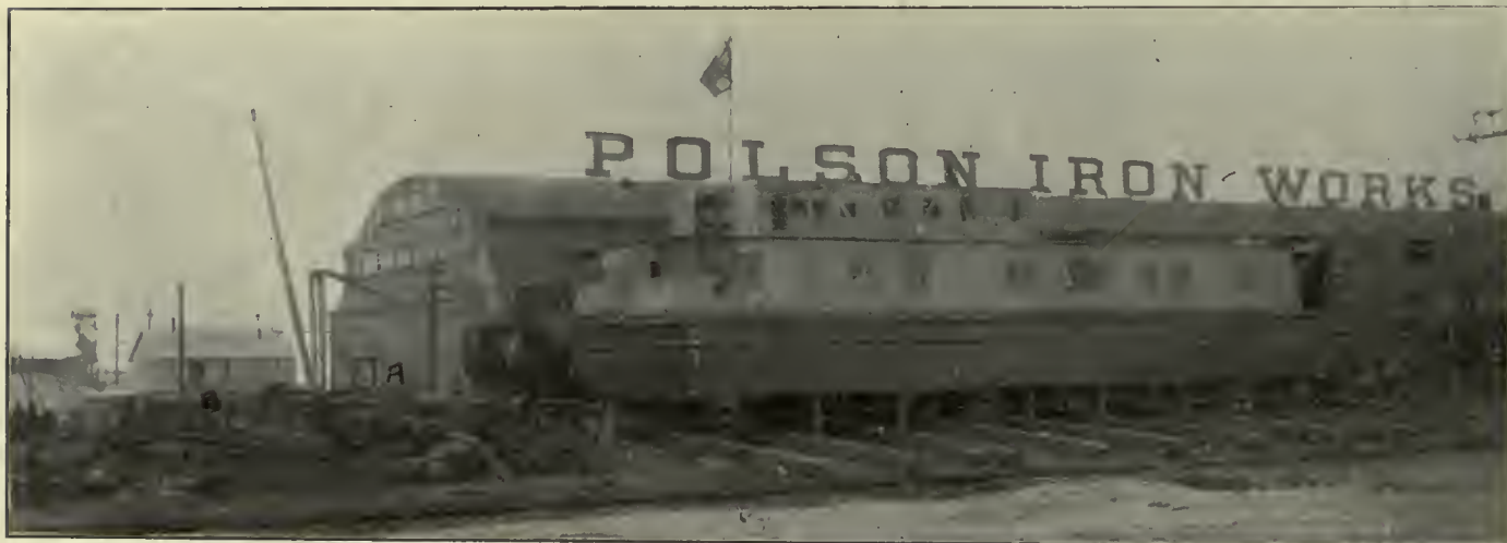
Fig. 1.—The Dredge Shuniah Before Launching, Polson Iron Works, Toronto.
