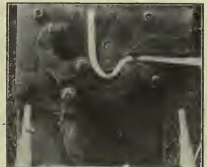
Fig. 6.—First Operation Bending Slice Bar Handle.
