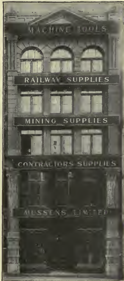
New Head Offices of Mussens Limited, Montreal.
