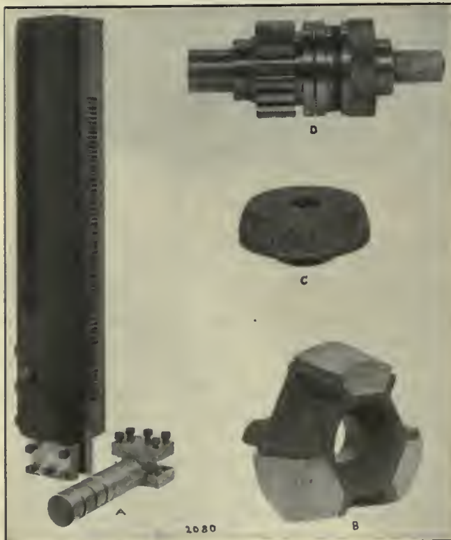
Fig. 3.—Details of New Model Boring and Turning Mills, Colburn Machine Tool Co.
