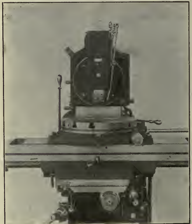
Slotting Attachment on Kearney & Trecker Milling Machine. Fig. 2.—Slotting Attachment on Kearney & Trecker's Milling Machine.
