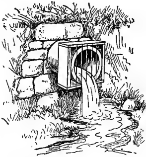
WATER ISSUING FROM AN UNDERGROUND DRAIN. 1
