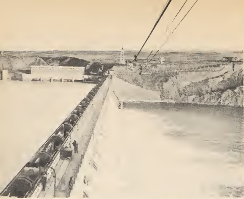
Irrigation dam on the Bow River near Bassano.
