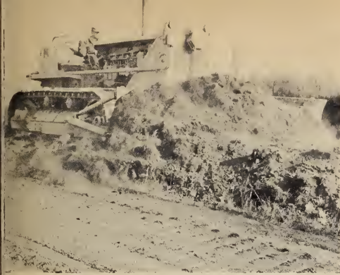
Municipal road-grading machinery in operation.
