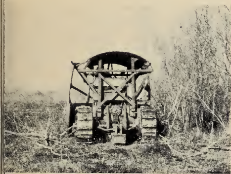
Clearing with modern equipment.
