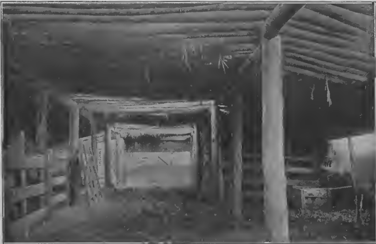
Interior of straw shed, 30 x 80 feet, IHC Farm, Grand Forks, N. D. Part of top has been thrown off. Note the subdividing panels.
