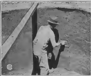
Plastering dirt with cement mortar.
