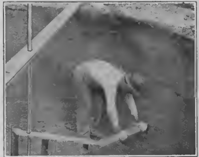
Reaming walls for plastering.
