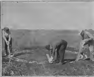
Marking out curb for pit silo.
