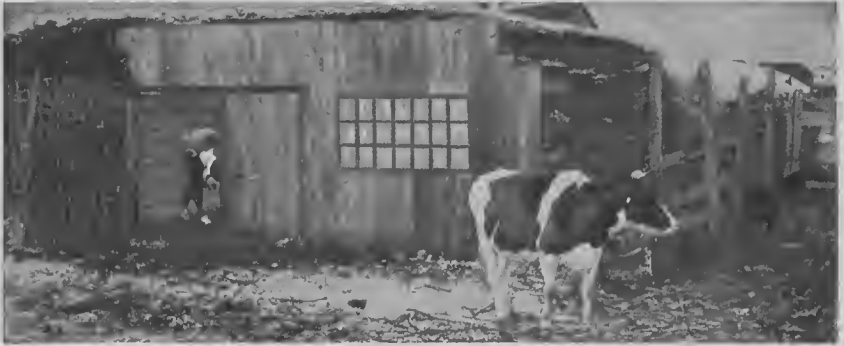
Note the sliding doors and the window on the end of the straw shed.
