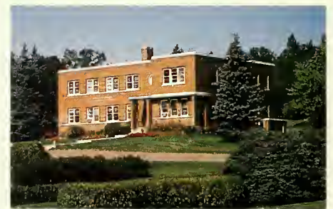
Main office, Brandon Research Station L'édifice principal de la Station de recherches de Brandon
