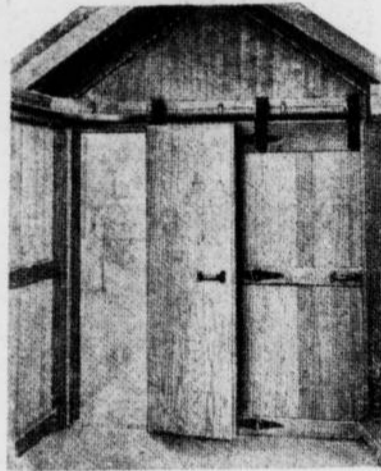
The Door is in three divisions, one of which swings on hinges.
