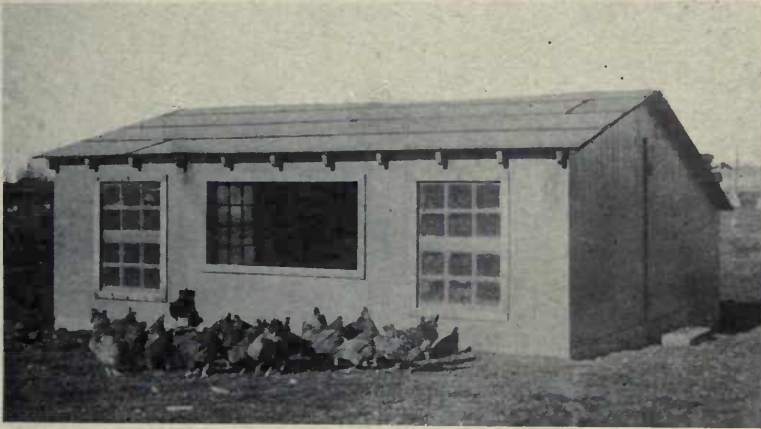
DEMONSTRATION HOUSE AT COOKSHIRE AND ROUGEMONT, QUE
