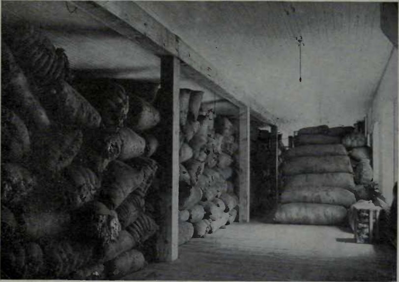
WOOL IN SACKS STORED AT THE DOMINION GOVERNMENT WOOL WAREHOUSE, TORONTO
