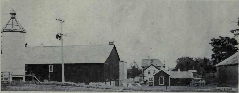
GENERAL VIEW OF FARM SERVED WITH HYDRO POWER, SHOWING FARM SERVICE TRANSFORMERS—SERVICE TO BARN AND HOUSE.
