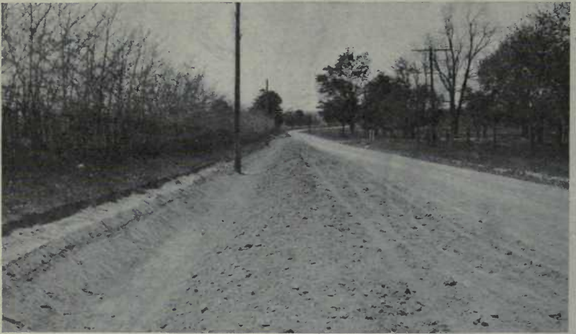
PROVINCIAL HIGHWAY GRAVEL ROAD WELL DITCHED AND GRADED.
