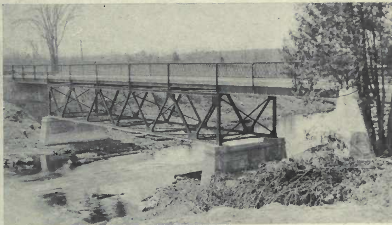
BRIDGE ON A LANARK COUNTY ROAD SUBSIDIZED BY THE PROVINCE.
