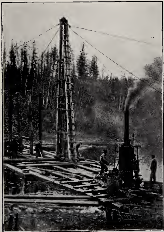
THE PILE-DRIVER AT WORK ON THE BRIDGE.
