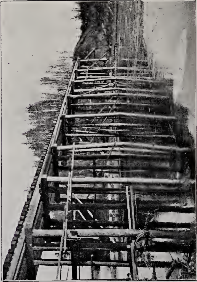
THE 200-FT. SPAN TRESTLE BRIDGE AT POST LAKE.
