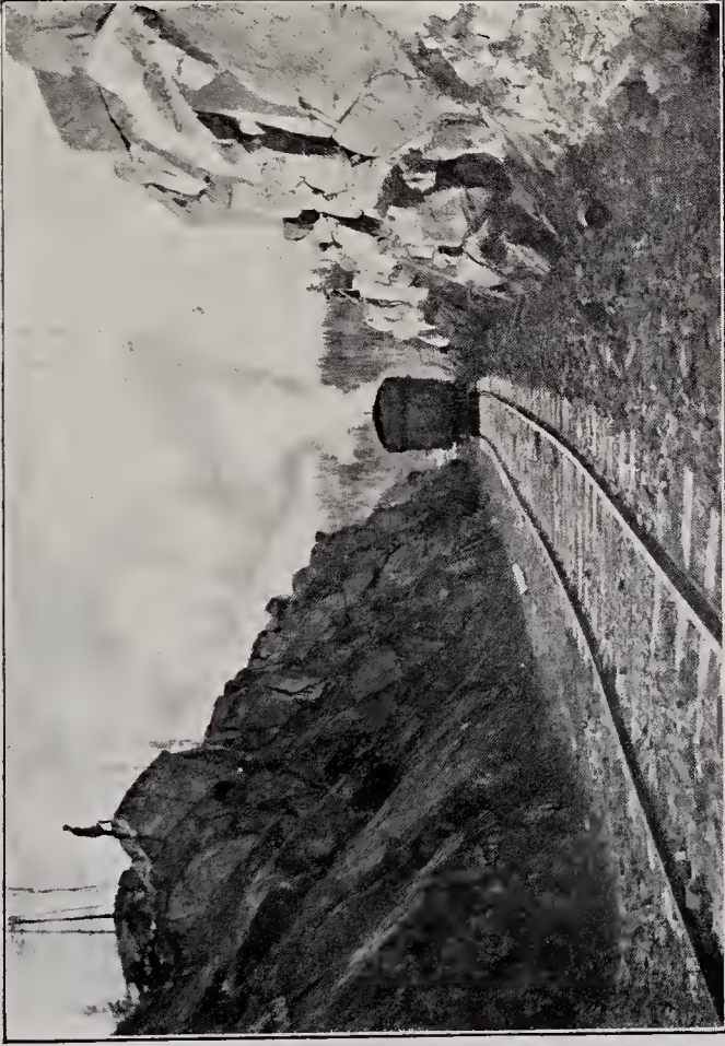
TRAIN PASSING THROUGH A ROCK CUTTING BEFORE THE TRACK WAS BALLASTED OR LINED-UP.
