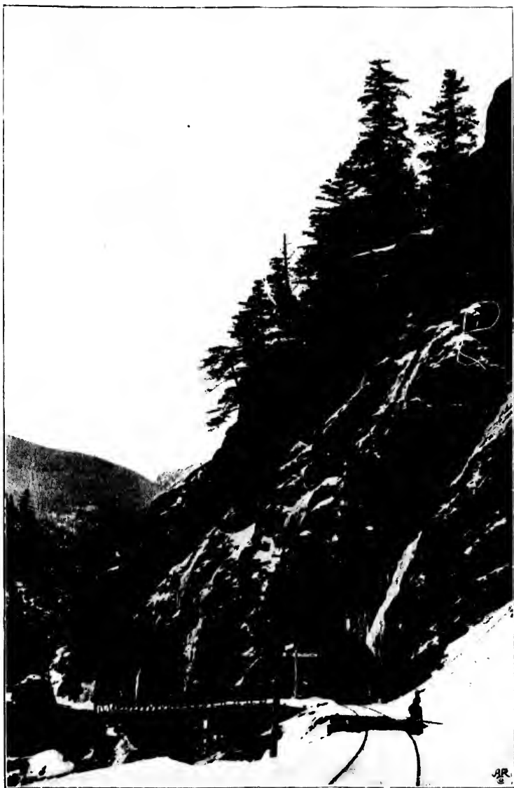
WAGON ROAD AROUND BLUFF—RAILWAY TUNNEL THROUGH IT.
