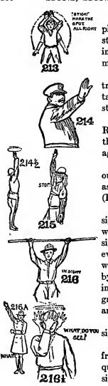
Fig. 213. You are at the right place—Mark it there—Hold your staff there. Signal used when placing a man in line usually the flagman. (Surveyors' signal.)
