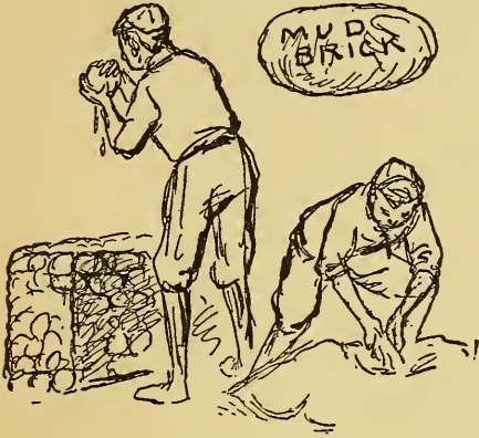
Fig. 138.—Making Mud Bricks
