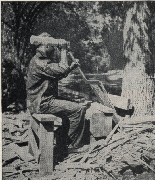
FIGURE 20.—Splitting shakes with the froe.
