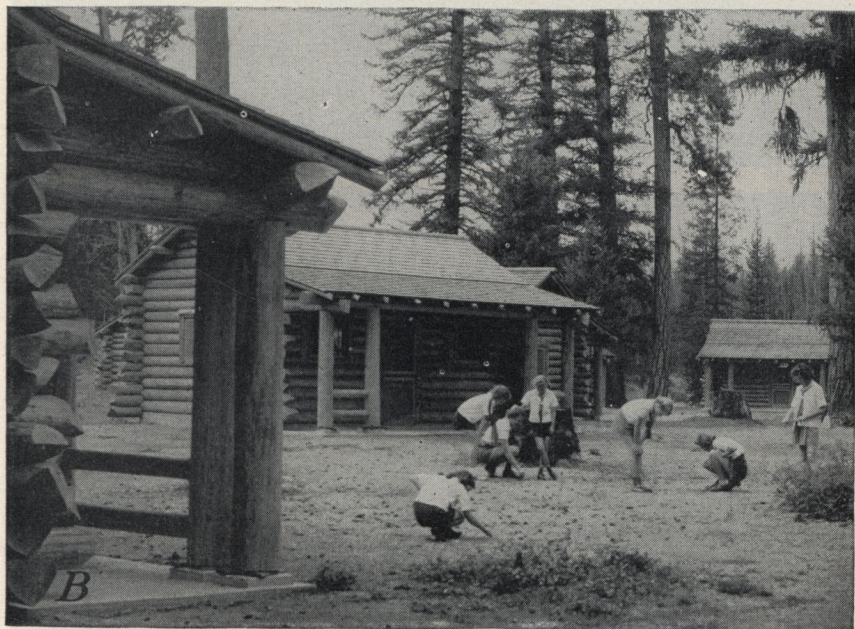
FIGURE 34.—Organization camp at Seely Lake showing log work in greater detail. A , Entrance wing; B , cabin group. Note the wedges under porch post to provide for settling of walls. Wedges are gradually driven out as necessary.
