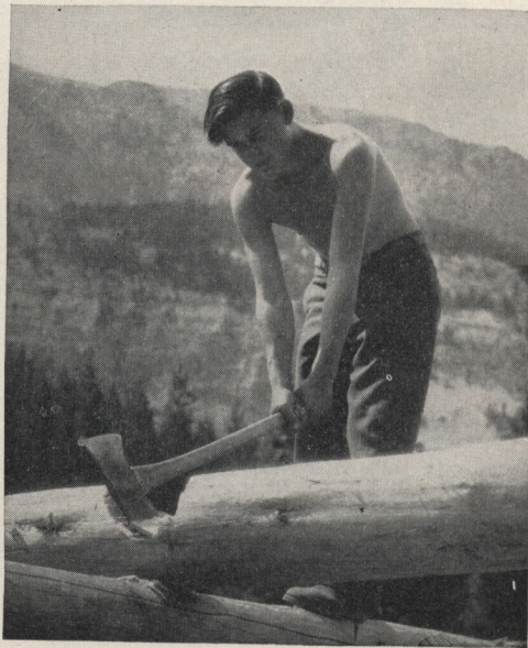
FIGURE 5.—Chopping the notch in a saddle corner.
