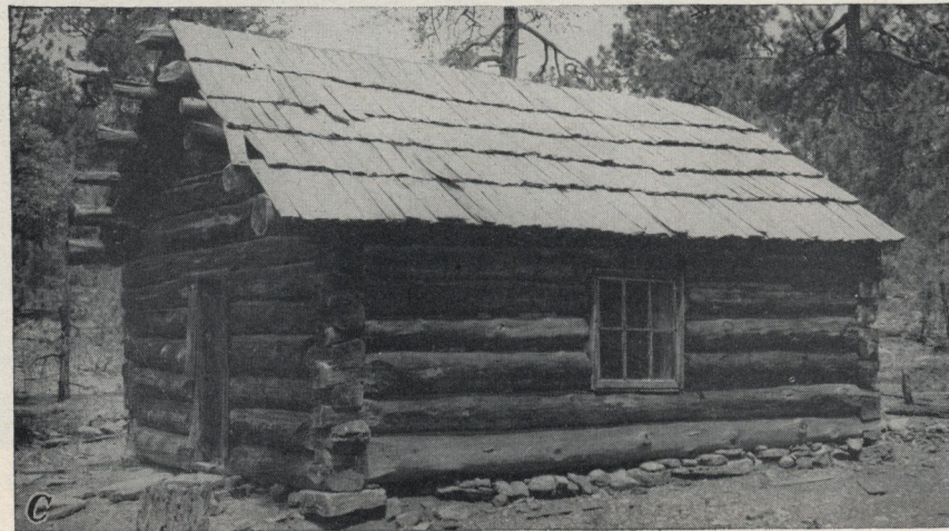
FIGURE 35.—Early types of log structures built by the U. S. Forest Service in the West. A, Ranger station, Gallatin National Forest, Mont.; B, ranger's dwelling, Nezperce National Forest, Idaho; C, log cabin in Arizona.
