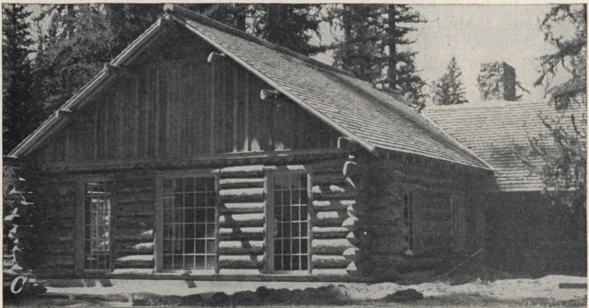
FIGURE 33.—Modern structures showing effective use of log construction in recreation buildings on national forests in Montana. A, Dude ranch; B and C, recreation buildings and mess hall, Seely Lake.
