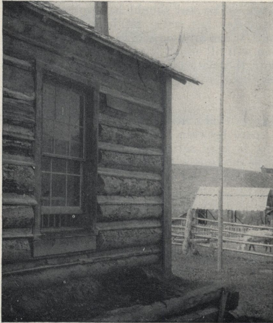
FIGURE 26.—Wood daubing strips.
