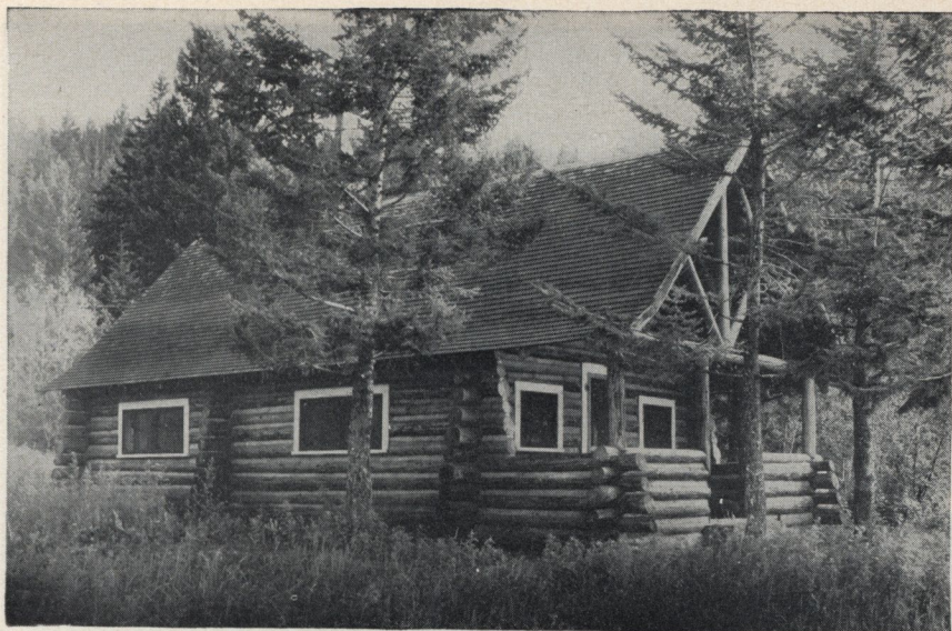
FIGURE 32.—A useful type of modern log dwelling—ranger station, Gallatin National Forest, Mont.
