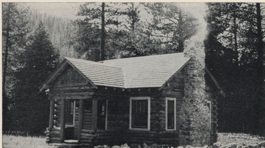
FIGURE 28.—Fine example of milled-log construction—ranger's dwelling, Whitman National Forest, Oreg.
