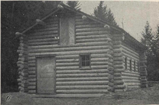
FIGURE 3.—Ranger station, Gallatin National Forest, Mont., illustrating effective use of round-notch corners. A, and B, Dwelling under construction; C, barn.
