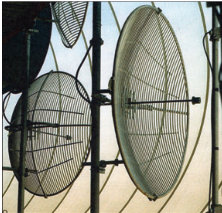
The microwave dishes on the CN Tower
