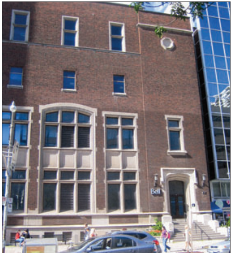
The Bell Building at 72 Eglinton Avenue East also as it now looks
