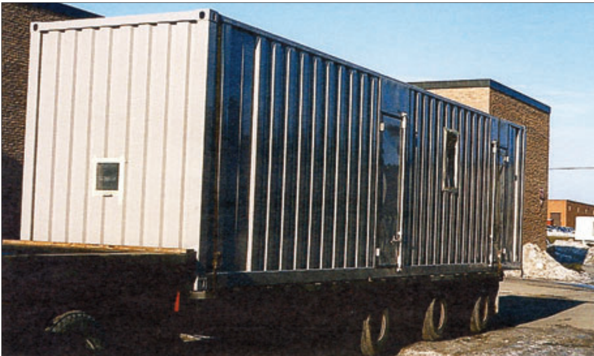
A Pre-Fab Cell site being delivered
