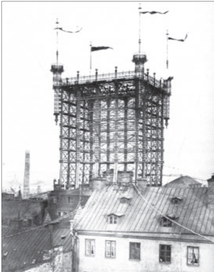
The great Telephone Tower, Stockholm, 1910
