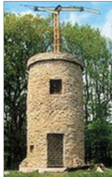
A replica of a Chappe Tower
