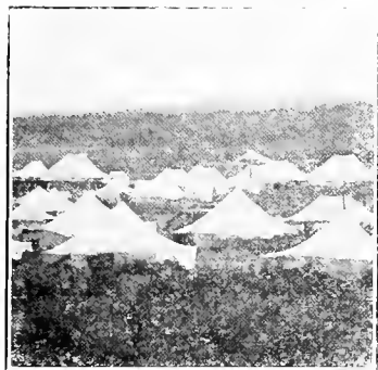
On railway construction, Western Canada, 1908.
