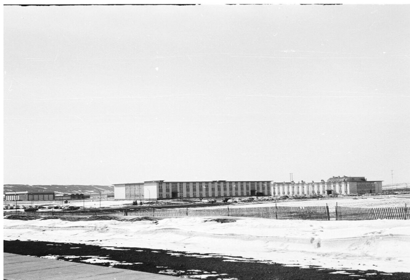
Figure 20.8: The University of Alberta at Calgary in 1962. In the far left background is the “gym”, with the original two-storey (plus basement) Arts and Sciences buildings at right angles to each other.
