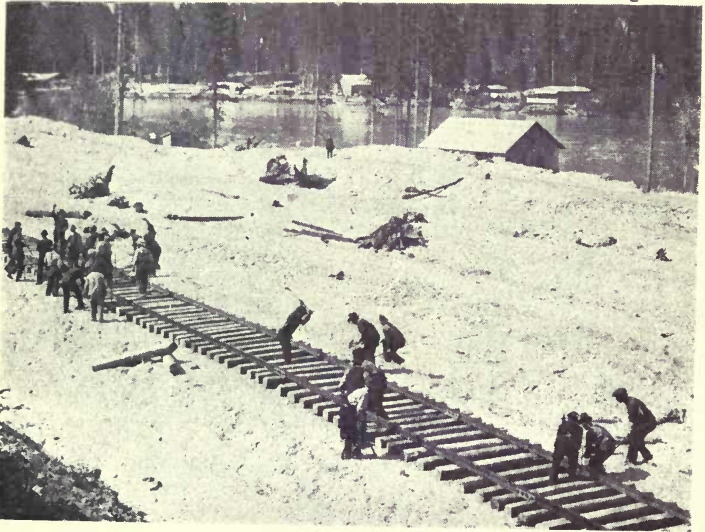
WITH THE LIFT-GANG.
