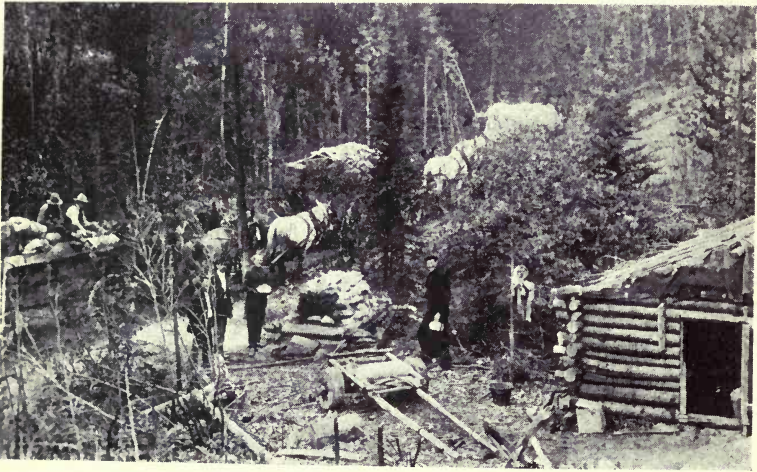
TOTING SUPPLIES FOR CONSTRUCTION IN THE ROCKIES.
