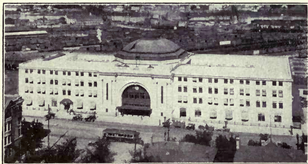
CANADIAN NATIONAL STATION, WINNIPEG.
