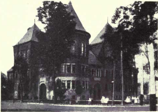
CENTRAL SCHOOL, CHATHAM, ONT.
