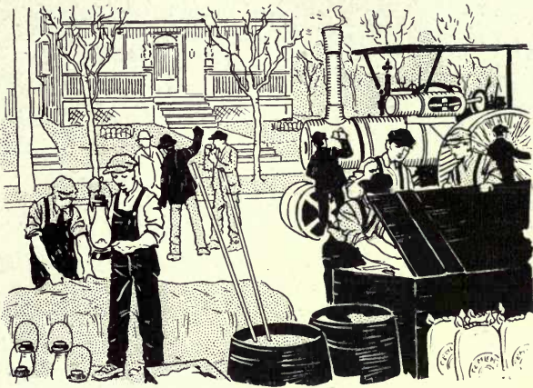
SIX O'CLOCK WITH A ROAD-MAKING GANG.
