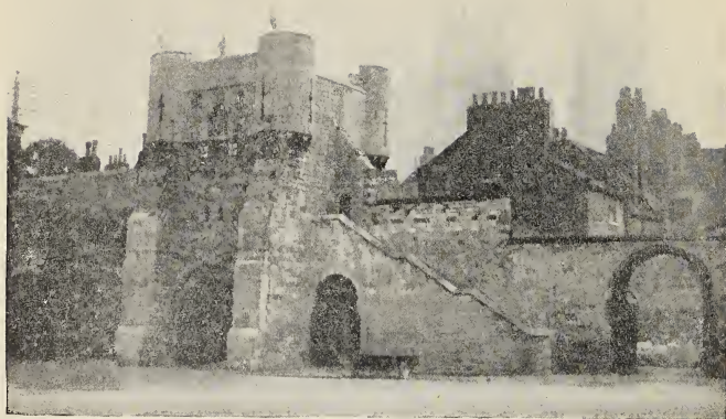
THE WALLS OF YORK
