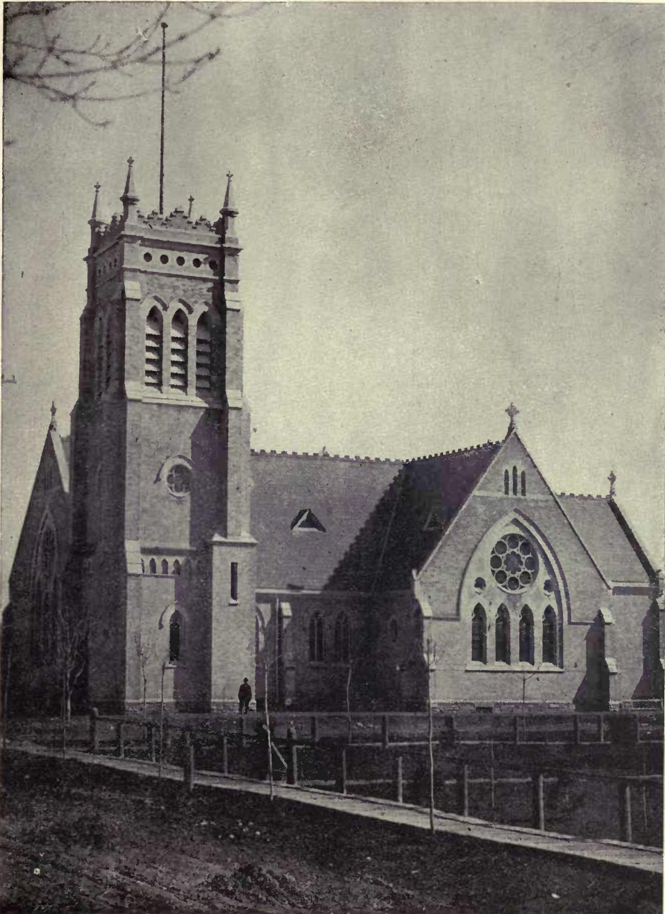
THE TRIVITT MEMORIAL CHURCH, EXETER, ONT. SOUTH SIDE VIEW. ENTRANCE ON THE NORTH SIDE.
