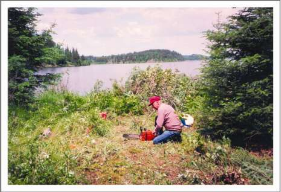
Douglas Barker helping in selecting and clearing building site. Two Loon Island – Summer 1994
