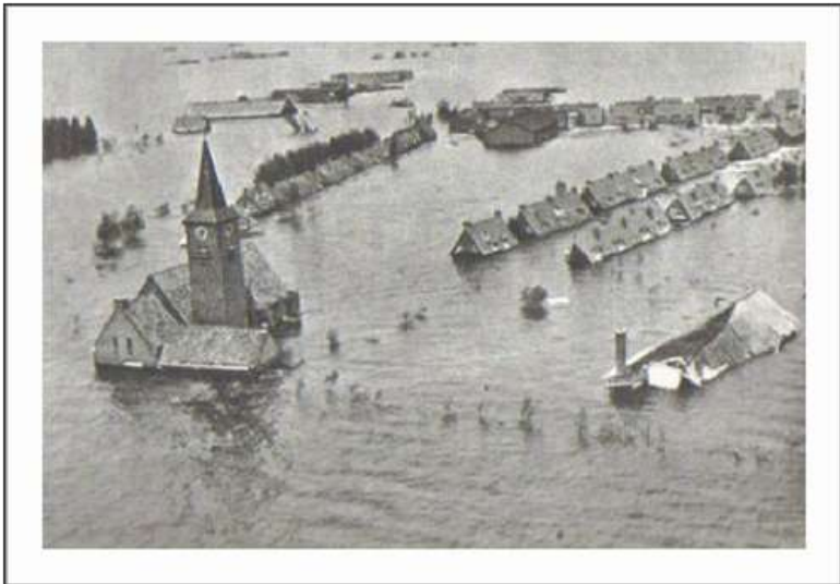
Fearing an invasion from the Zuiderzee, the Germans flooded the prosperous villages of the newly claimed Wieringermeer Polder.
