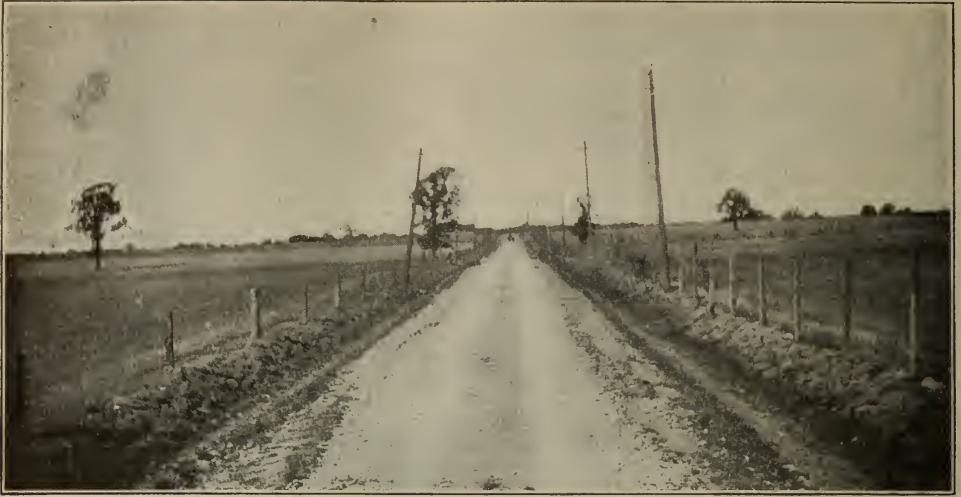
A road in Eastern Ontario, through a low tract of country, well drained and surfaced.
