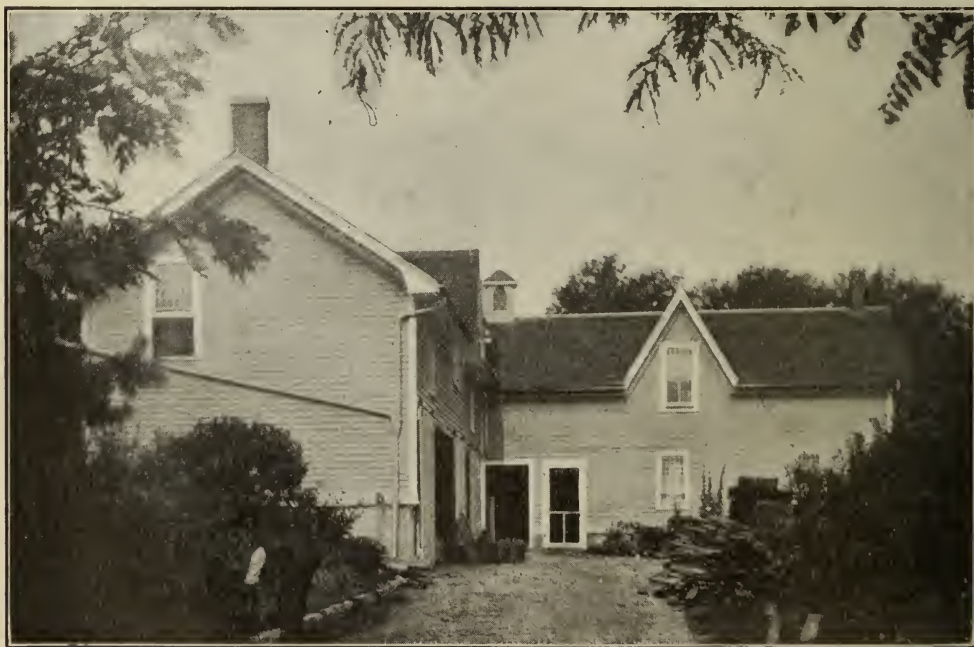
This is F. L. Green's farm dairy building, Ontario Co. A complete system of farm lighting and power is furnished from a dynamo installed in his grist mill nearby and run by water power. His costs for electrical operation are decidedly cheap.
