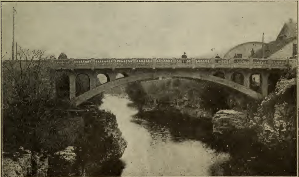
A single arch concrete bridge, County of Wellington. The rock formation is especially adapted to this type of structure.
