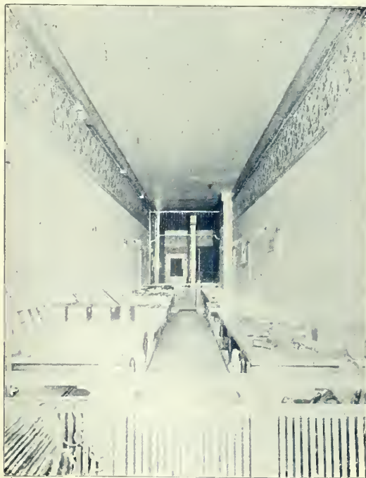
Luxfer Prisms successfully lighting store 100 feet long.
