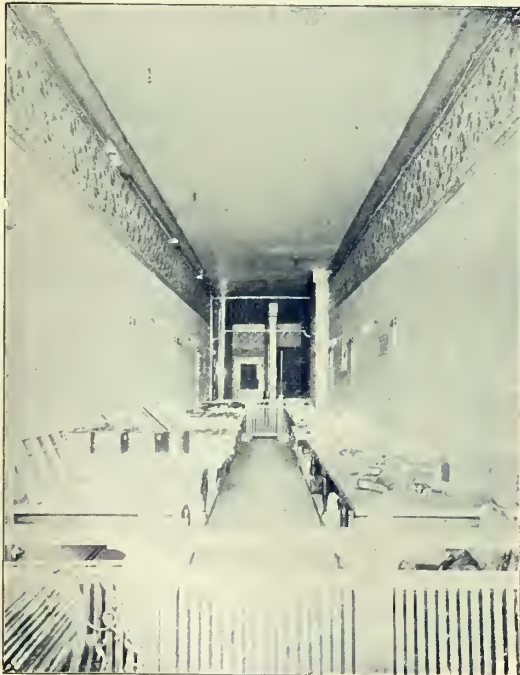
Luxfer Prisms successfully lighting store 100 feet long.
