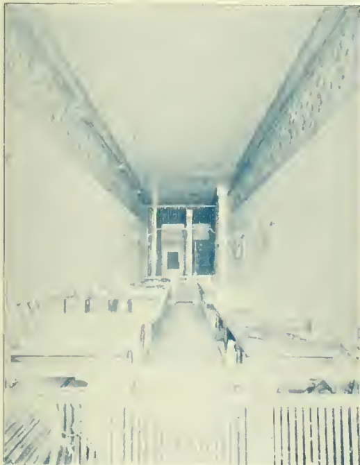
Luxfer Prisms successfully lighting a store 100 feet long.
