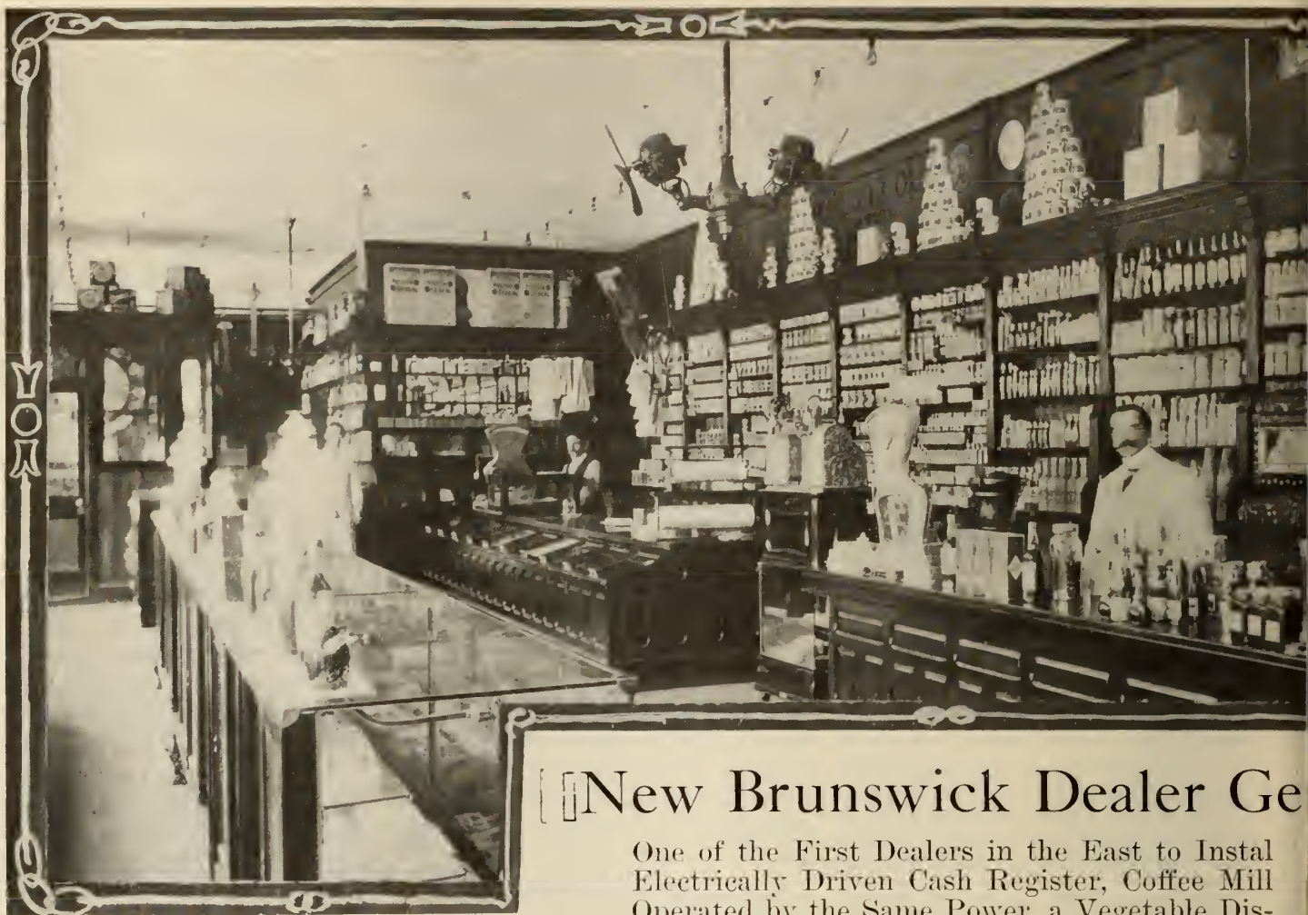
Interior of the Philips store in St. John, N.B., with counters, show cases, cash register with lead-glass case beneath, offices in rear, two double electric fans, etc.
