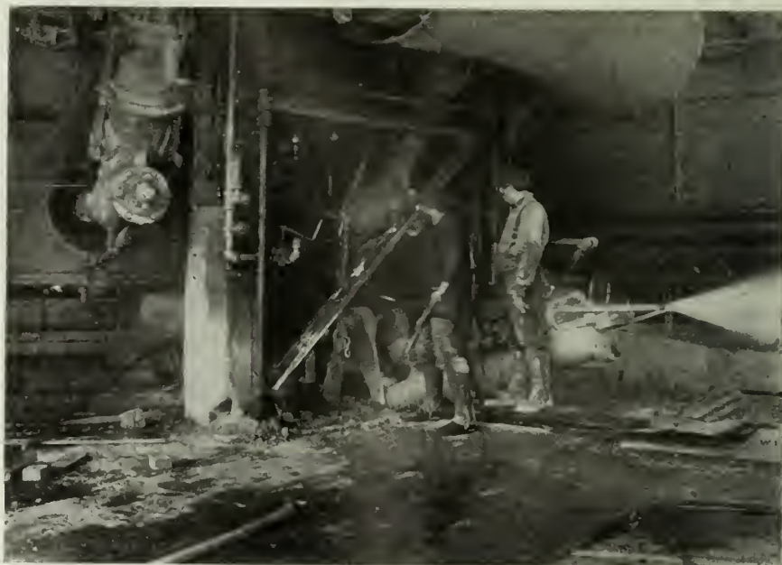
FIG. 18. SAFE WAY TO STOP TAPPING HOLE. Helper is using shovel and standing away from the trough and the tapping hole.
