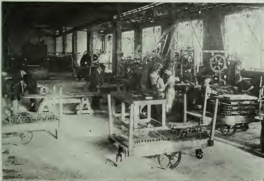
COMPONENT PARTS OF AUTOMOBILE FRAMES IN PROCESS OF MANUFACTURE IN FRAME DEPARTMENT.
