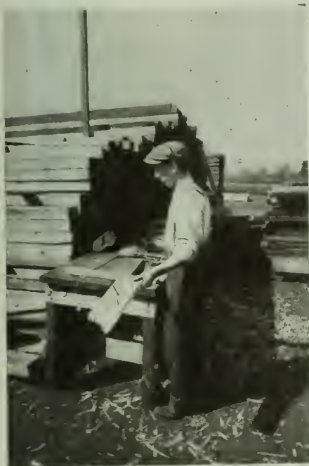
FIG. 38. WORKMAN THROWS DOWN BOARD WITH NAILS IN IT.
