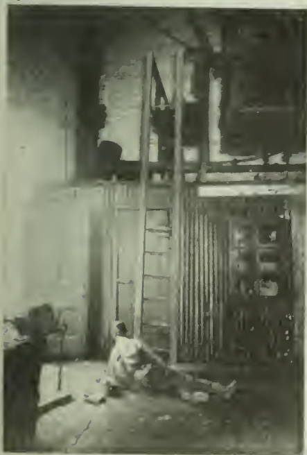
FIG. 9 MAN FALLS FROM LADDER
