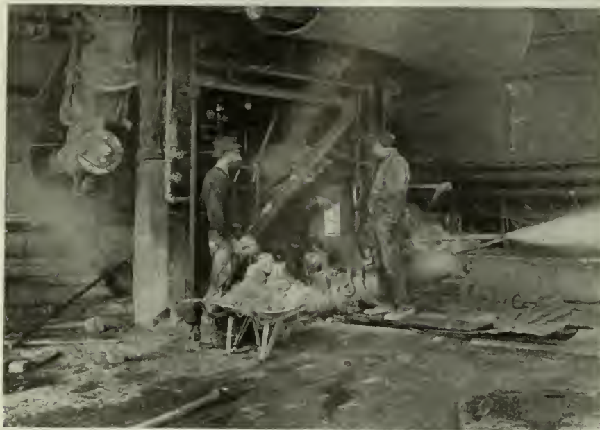
FIG. 17. UNSAFE WAY TO STOP TAPPING HOLE. Helper is using his hands and standing too near tapping hole.
