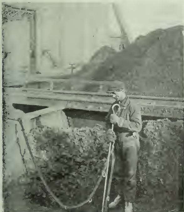
FIG. 25. PROPER EQUIPMENT FOR MAN WORKING IN ORE BIN. NOTE LIFE LINE ATTACHED TO HIS BODY AND TO CROSS BEAM OF BIN.
