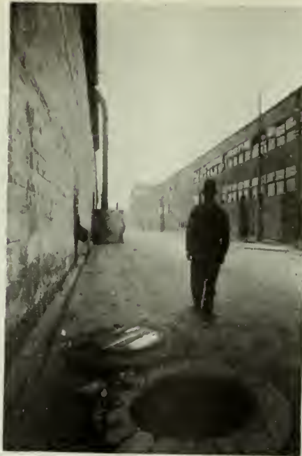
FIG. 28—WORKMAN LEAVING MANHOLE UNCOVERED
