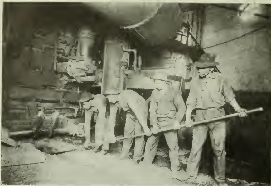
FIG. 13. UNSAFE METHOD OF DRILLING A TAPPING HOLE.
