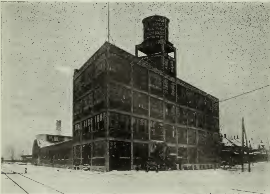
MAIN BUILDING OF PLANT NO. 1. WHERE HEAD OFFICE OF COMPANY IS LOCATED.
