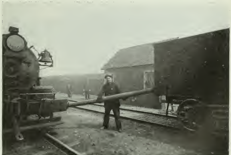
FIG. 21. SAFEST WAY OF USING POLE TO PLACE CARS.
