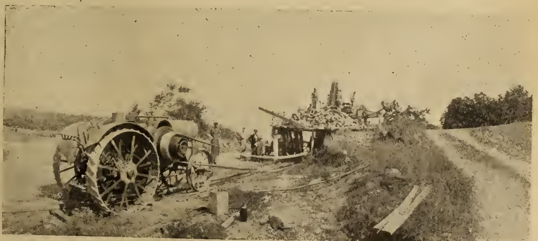
Tractor on belt work operating a stone crusher.
