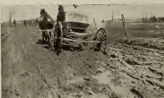
They're getting busy here—making a rock fill to widen the road-bed.
