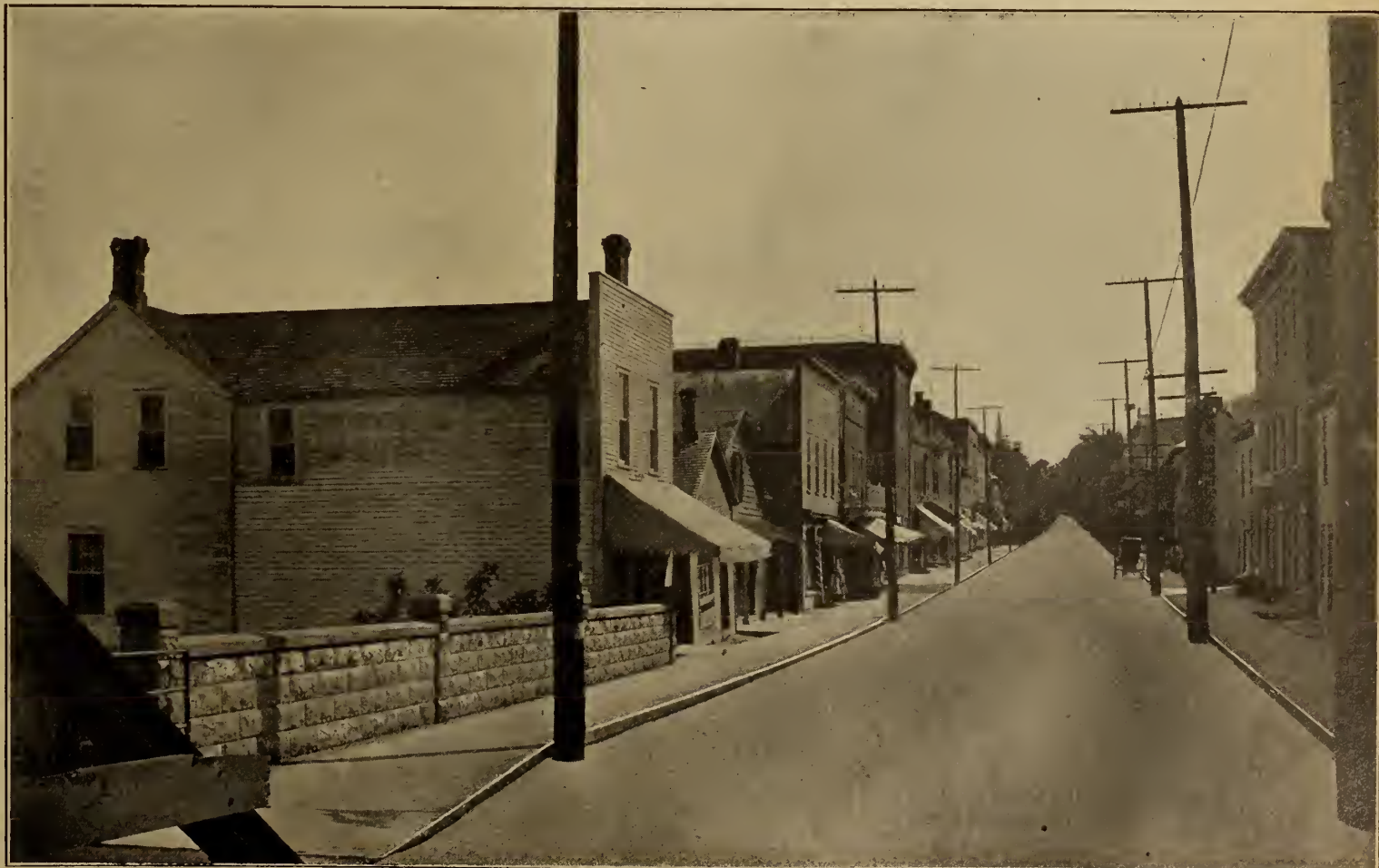
A section of the concrete roadway built by the Dominion Concrete Co. for the Town of Kemptville.
