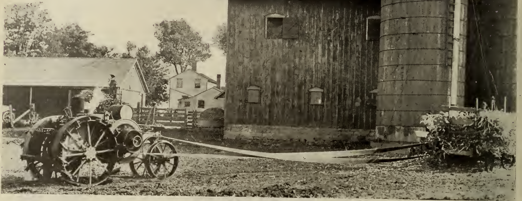
The tractor on belt work filling a silo.
