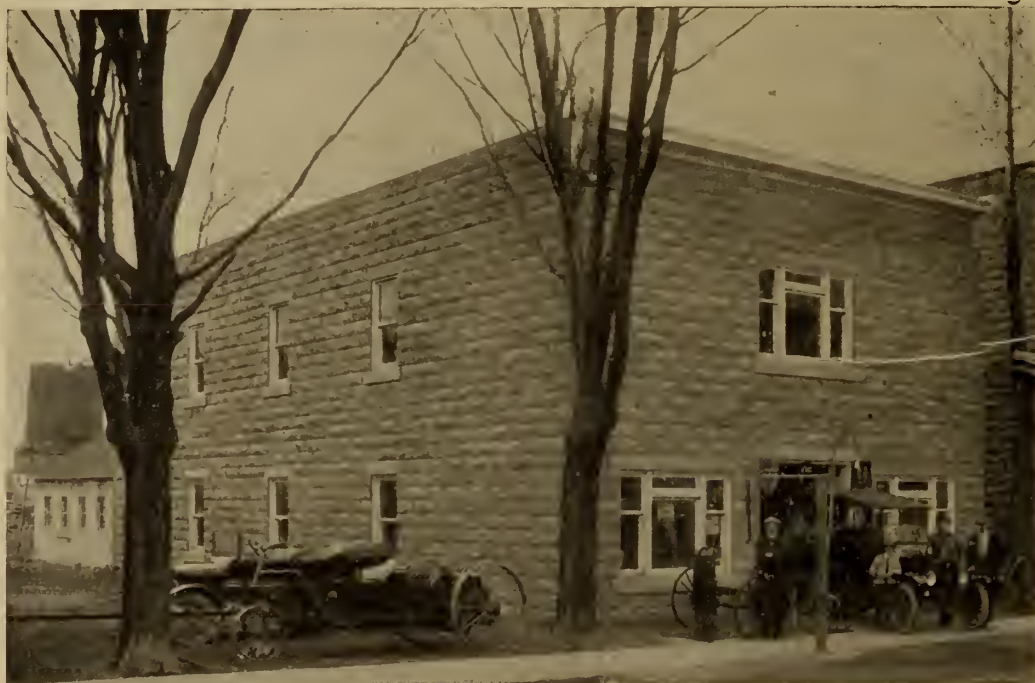
Anderson-Langstaff Garage, showing line up of cars and implements.
