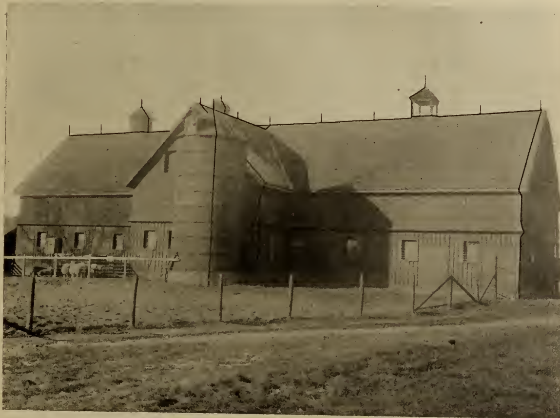
Sheep Building, Central Experimental Farm, Ottawa, protected with cable and fixtures.
