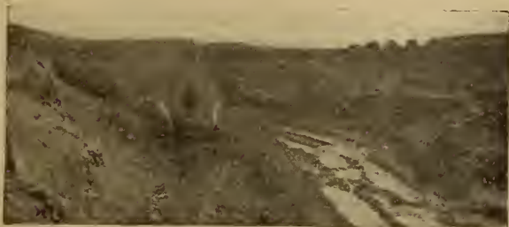
One of the Harvester Company's large open pit mines.
