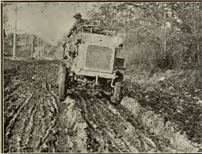
Showing how Trucks may be used on bad roads.
