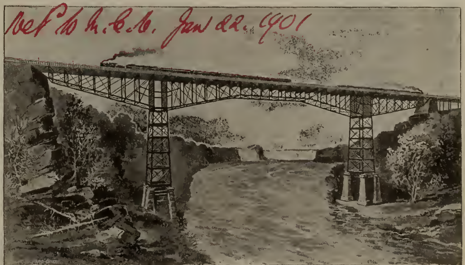
MICHIGAN CENTRAL RY. CANTILEVER BRIDGE, NIAGARA FALLS, ONT.
