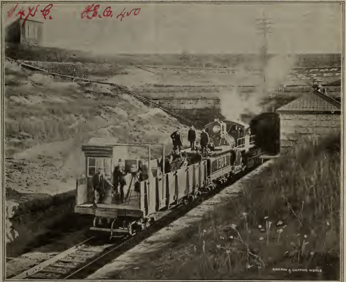
OUTFIT USED IN TAKING FLASHLIGHT PHOTOGRAPH OF INTERIOR OF ST. CLAIR TUNNEL, GRAND TRUNK RAILWAY SYSTEM. SEE PAGE 15.
