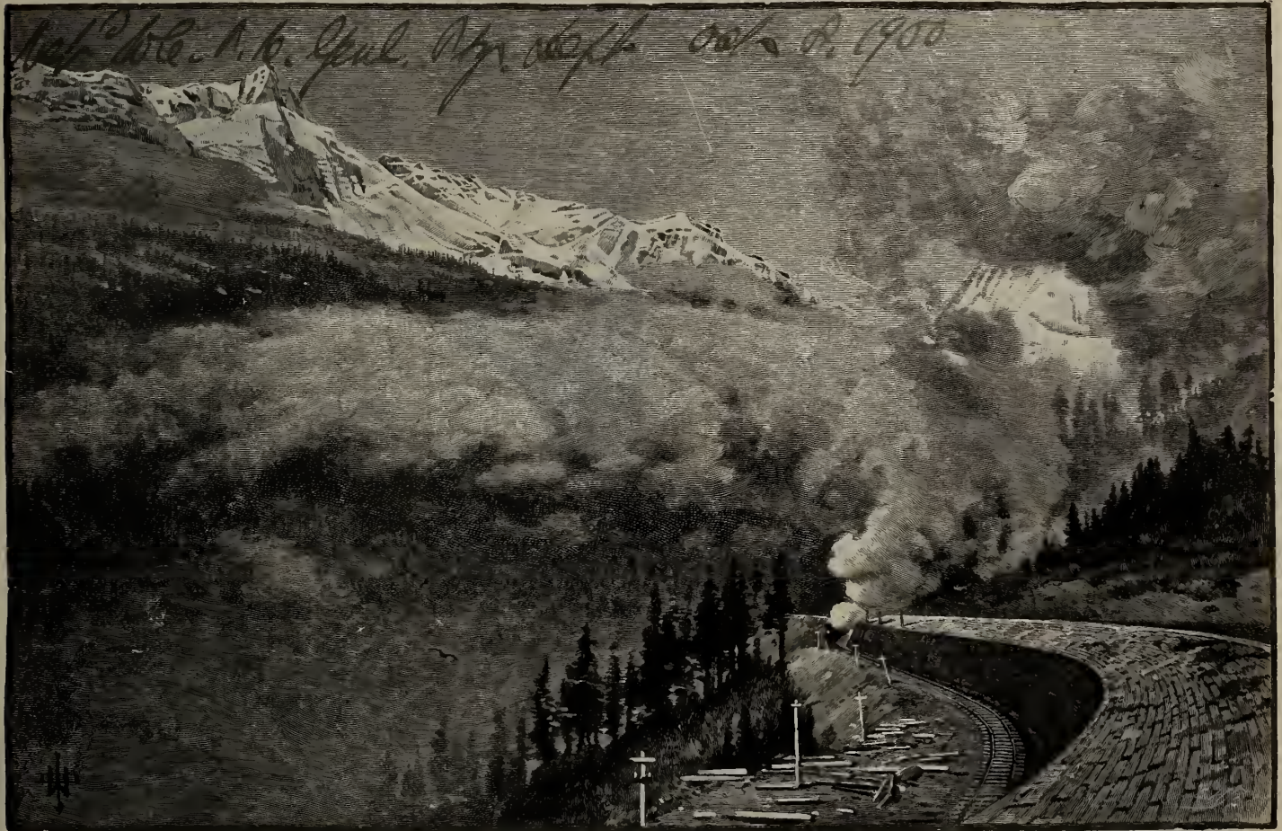
FIGURE 10.—SNOW-SHEDS ON THE C. P. R. IN THE SELKIRK MOUNTAINS, B. C. THE WINTER TRACK UNDER COVER ; THE OUTER TRACK FOR SUMMER USE. (SEE PAGE 258.)
