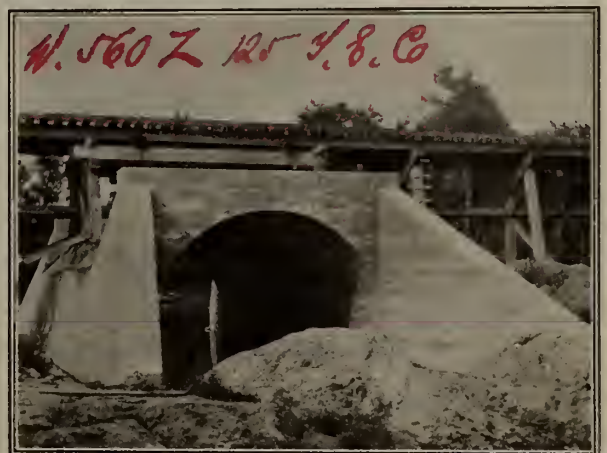
END VIEW OF CULVERT AND WINGWALLS, L. E. AND D. R. RY.
