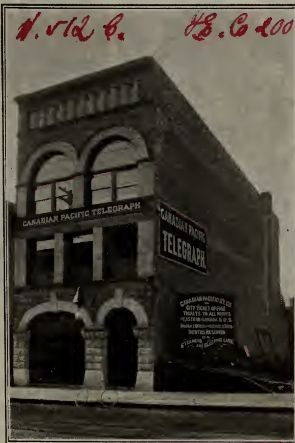
C.P.R. TELEGRAPH BUILDING, VANCOUVER.
