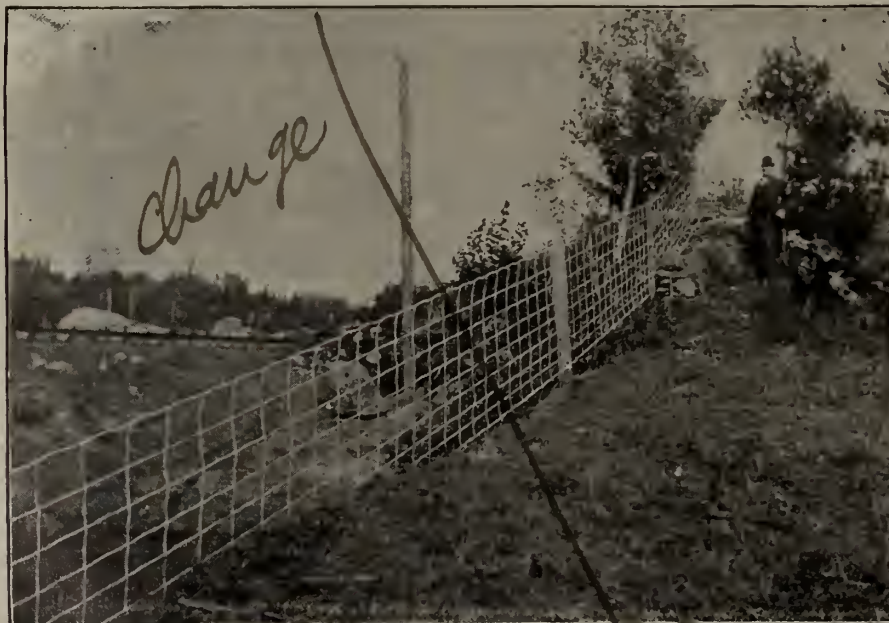
Page Fencing on Pembroke Southern Railway.
