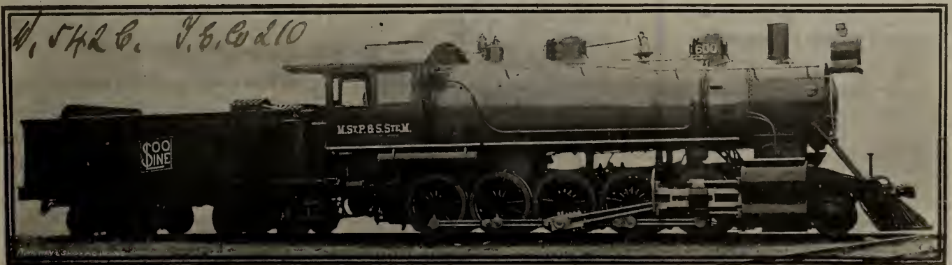
BALDWIN COMPOUND DECAPOD LOCOMOTIVE FOR MINNEAPOLIS, ST. PAUL AND SAULT STE. MARIE RAILWAY.
