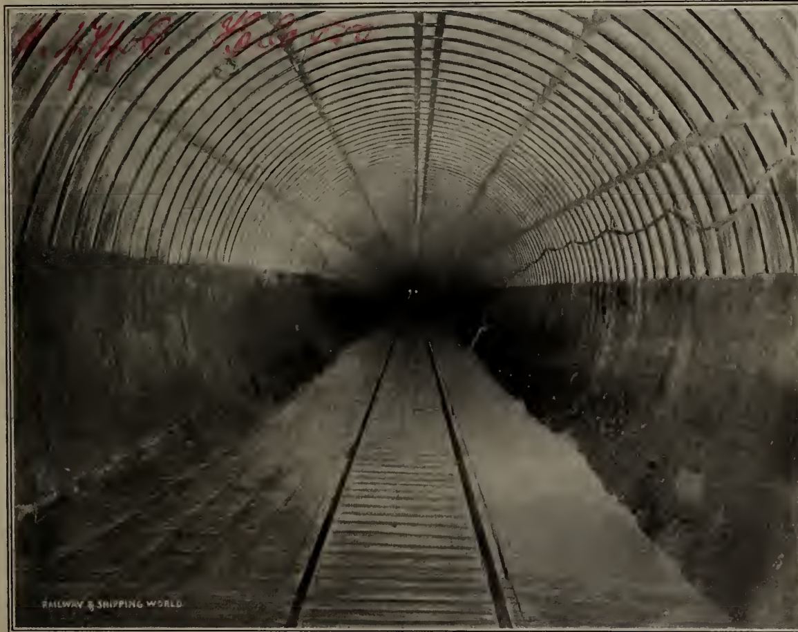
FLASH LIGHT PHOTOGRAPH OF INTERIOR OF ST. CLAIR TUNNEL GRAND TRUNK RAILWAY SYSTEM.
