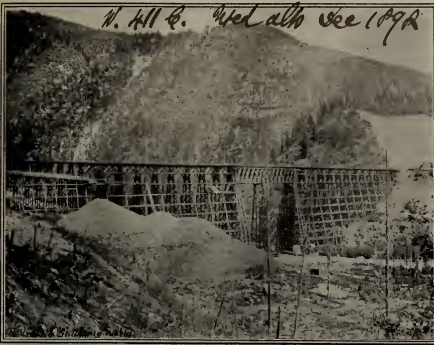
FIGURE 8.—HYDRAULIC FILLING ON THE C.P.R. AT MOUNTAIN CREEK, B.C. (SEE PAGE 261.)
