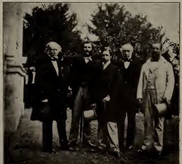
H. R. H. THE PRINCE OF WALES AND SUITE PRESENT AT OPENING OF VICTORIA TUBULAR BRIDGE, 1860.
