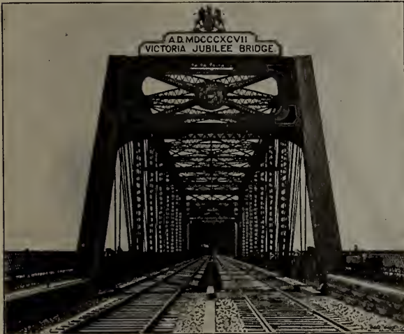
PORTAL VICTORIA JUBILEE BRIDGE.
