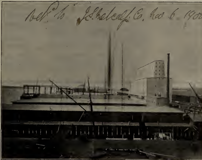
GRAND TRUNK RAILWAY ELEVATOR AT PORTLAND, MAINE.
