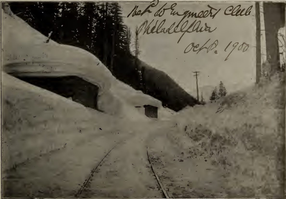
FIGURE 4.—A SNOW-CUT SHOWING DEPTH OF SNOW ON THE C. P. R., IN THE SELKIRK MOUNTAINS, B. C. (SEE PAGE 258.)
