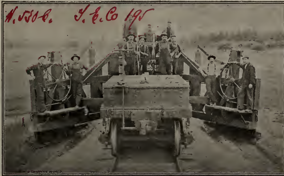
BOSTON AND MAINE SHOULDERING CAR IN SERVICE. FIGURE 3.
