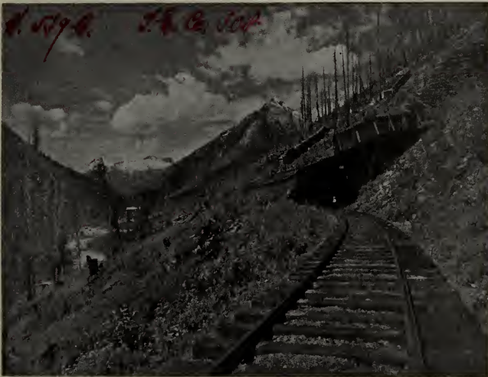
FIGURE 6.—A TYPICAL SNOW-SHED ON THE CANADIAN PACIFIC RAILWAY. (SEE PG. 259.)
