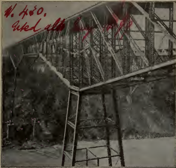
MICHIGAN CENTRAL RY. CANTILEVER BRIDGE, NIAGARA FALLS, ONT.
