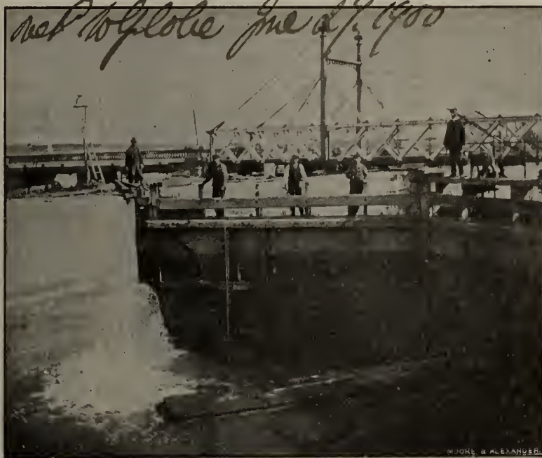
UPPER GATES ON LOCK 24, NEW WELLAND CANAL, THE SCENE OF THE DYNAMITE OUTRAGE ON APRIL 21, SHOWING WATER RUSHING THROUGH THE BREACH CAUSED BY THE DYNAMITE, AND REPAIRS COMMENCED.
