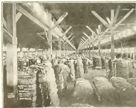
Warehouse 1,700 ft. long, 150 ft. wide.
