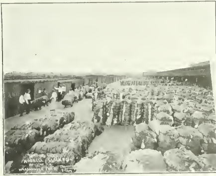
Loading Scene, Warehouse and Yard.
