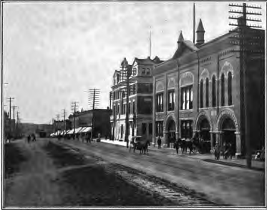
NEW WESTMINSTER IS NOT NOW THE SEAT OF PROVINCIAL GOVERNMENT BUT IS NEVERTHELESS A PROMISING CITY. THE CIVIC AND DOMINION GOVERNMENT BUILDINGS ARE SHOWN HERE
