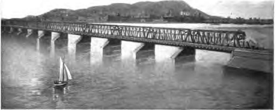
VICTORIA JUBILEE BRIDGE ACROSS THE ST. LAWRENCE RIVER, MONTREAL. BUILT ON THE SAME PIERS AS THE OLD VICTORIA TUBULAR BRIDGE. OPENED FOR TRAFFIC 1898.
