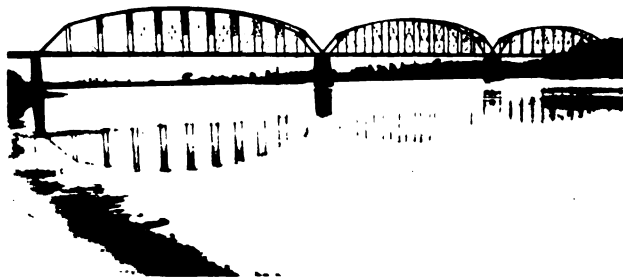
THE SOUTH BRIDGE AT CORNWALL ISLAND
