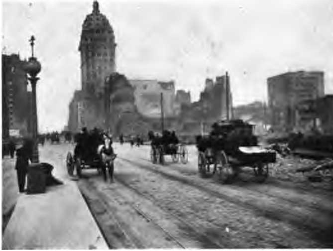
MARKET ST. AND THE "CALL" BUILDING AFTER BEING SWEEPED BY THE FIRE. THIS WAS THE HEART OF THE BUSINESS DISTRICT
