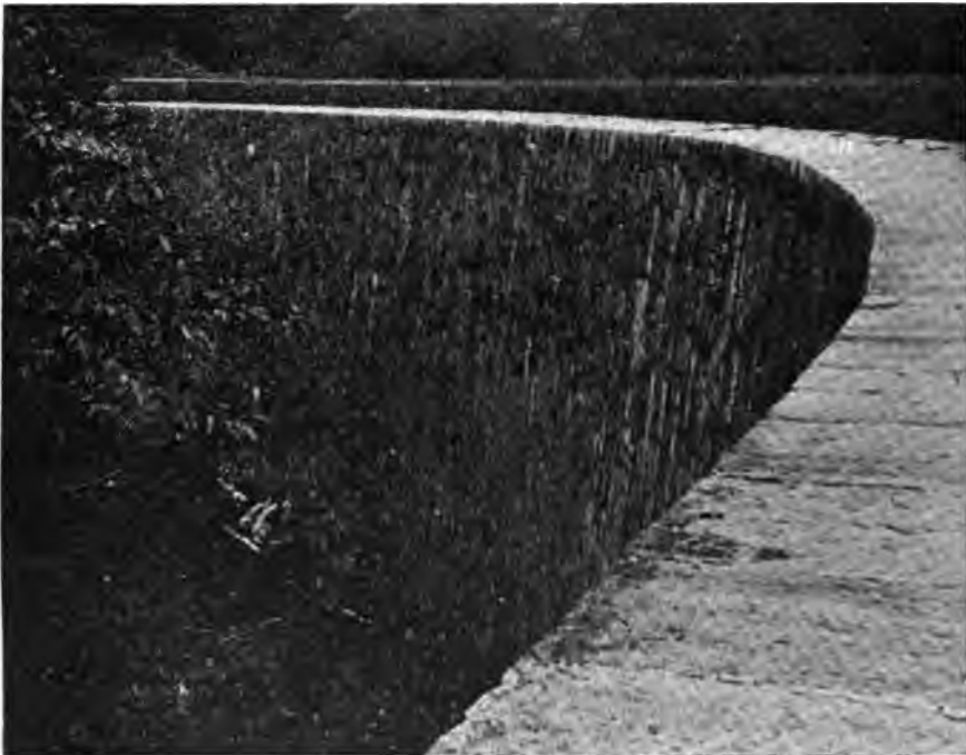
THE CURVED DAM AT SAND LAKE, JONES' FALLS
