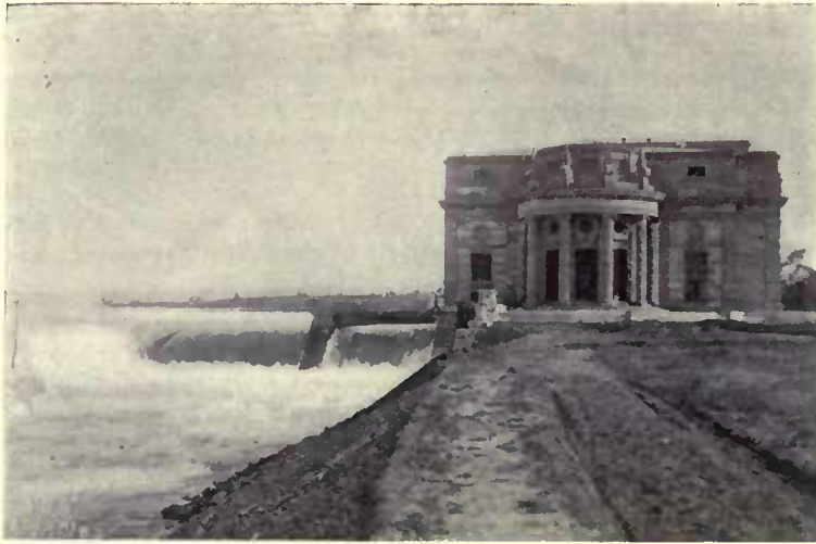
End view of Power House, Electrical Development Company, Niagara Falls, Ontario.
