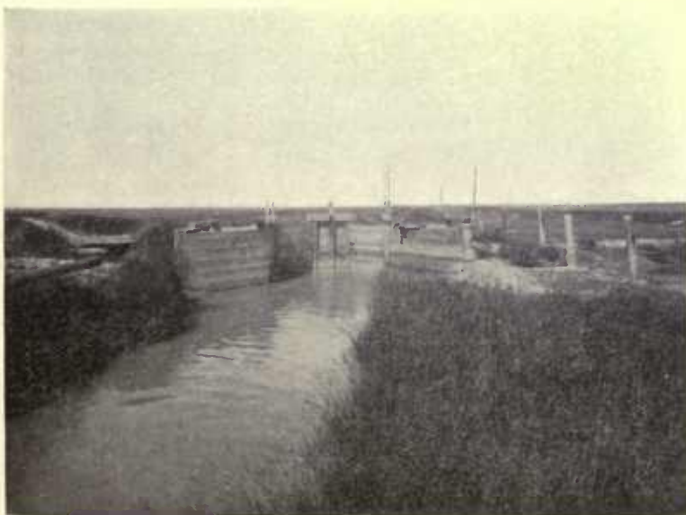
Headgates on the Galt Canal near Lethbridge, showing how the flow of water is controlled.
