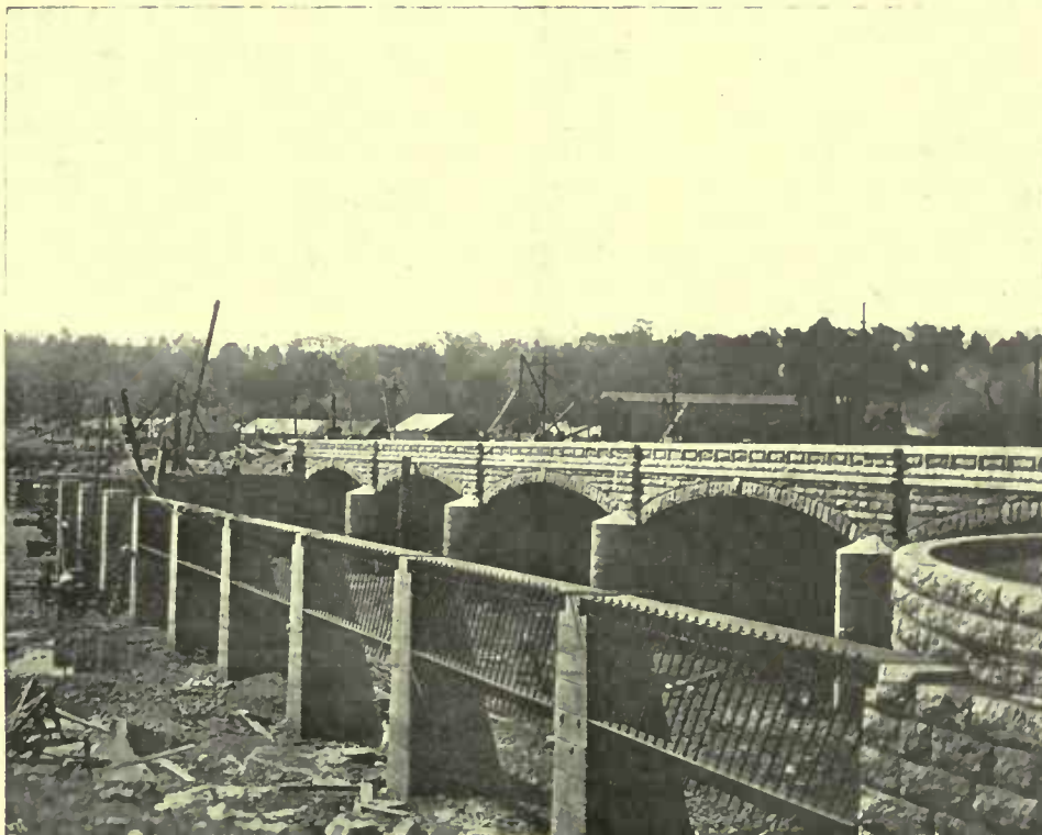
The Canadian Niagara Power Company's head works, showing the racks that prevent the ice from passing to the intake canal.
