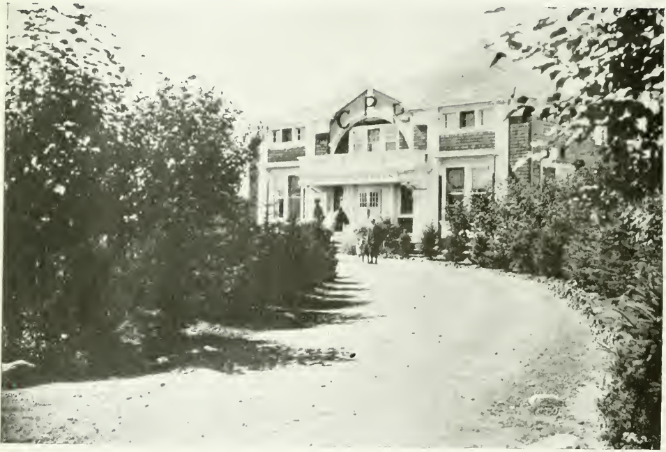
The planted approach to the C.P.R. Irrigation Offices.
