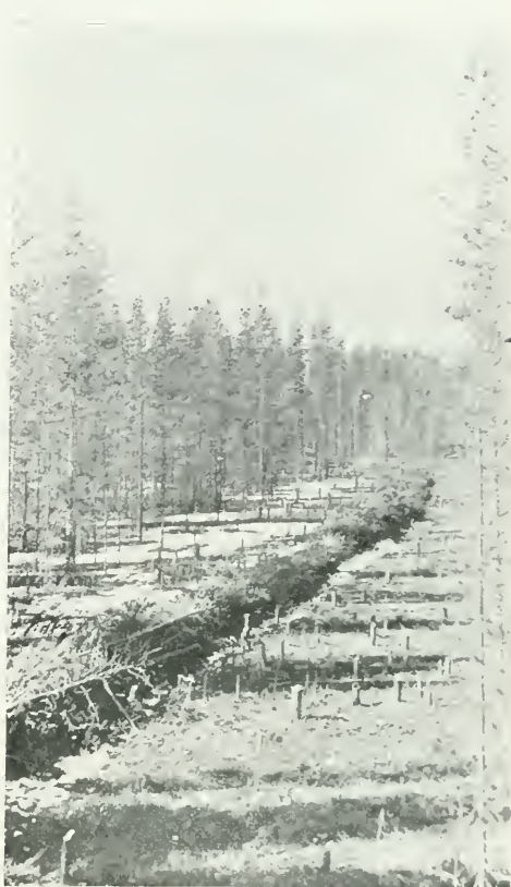
CUTTING A NEW ROAD IN BRITISH COLUMBIA Note how carefully the debris is piled for burning in the centre.
