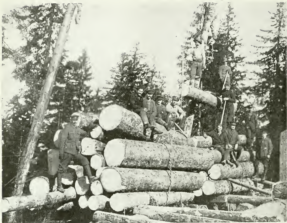
The Loading Deck at 60th Company Camp, Canadian Forestry Battalion, Vosges Mountains, France. The logs are fir and spruce.
