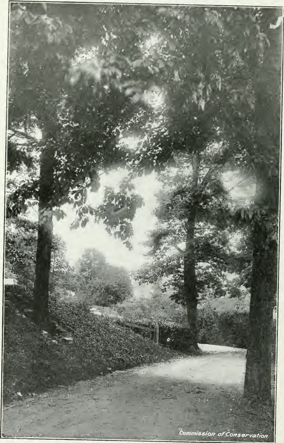
How a road can be cut through a woods without destroying the trees.
