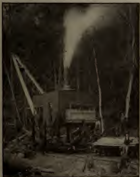
W. VIRGINIA: THE DECKER LOG LOADER, A SELF PROPELLING STEAM LOADER DESIGNED FOR SPECIAL CONDITIONS.
