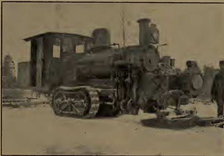
STEAM LOG HAULER USED IN MINNESOTA.
