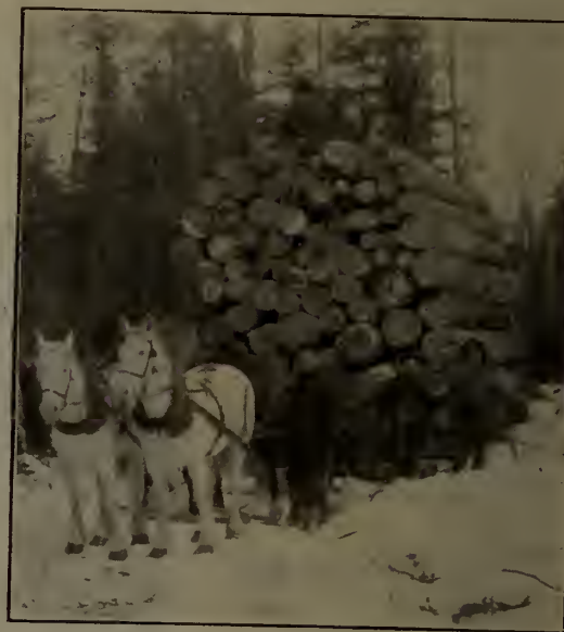
LOAD AT GRAHAM & HORNE'S CAMP, RAINY RIVER.—101 LOGS.
