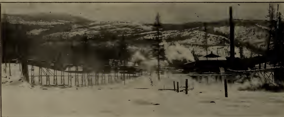
MOYIE LUMBER AND MILLING COMPANY—END VIEW OF MILL, SHOWING BOILER HOUSE, JACK LADDER, REFUSE CONVEYOR, BLOW PIPE AND PART OF MILL POND.
