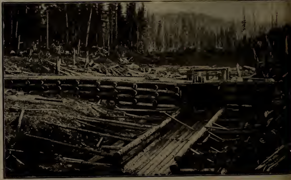
DAM ON THREE VALLEY CREEK, USED FOR COLLECTING LOGS AND RAISING A HEAD OF WATER TO CARRY LOGS DOWN CREEK.
