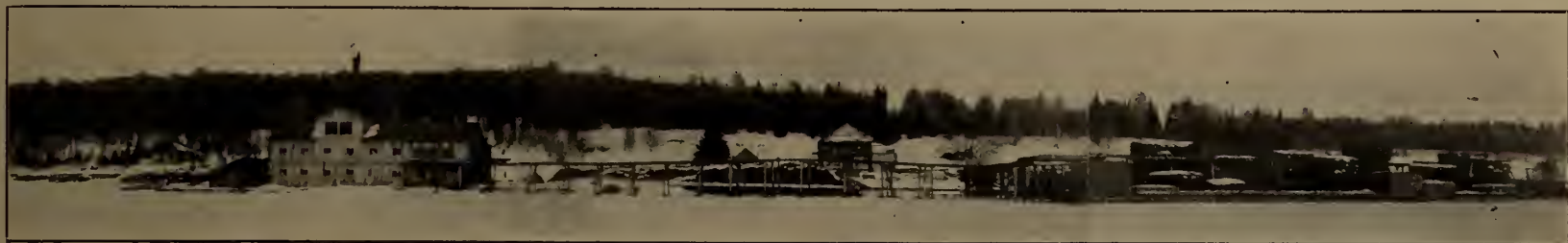
NEW MILL OF THE J. E. MURPHY LUMBER COMPANY AT MILFORD HAVEN, ONT.
