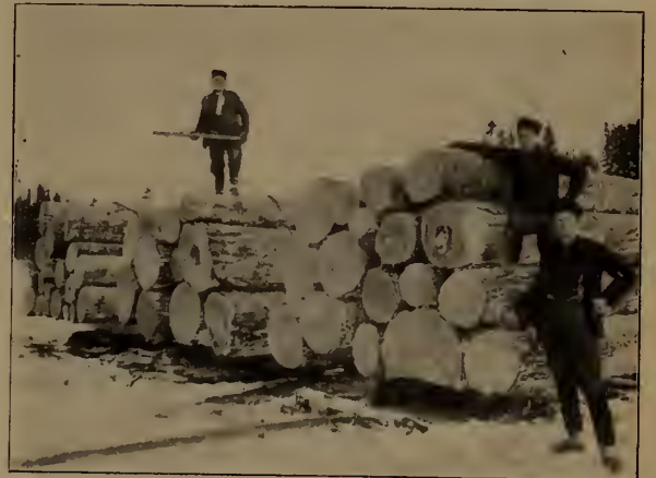
LOGS READY FOR THE MORNING, ARDILL'S CAMP, GILLIES BROS. COMPANY, COULONGE.
