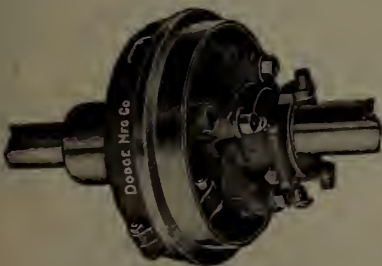
Friction Coupling.
