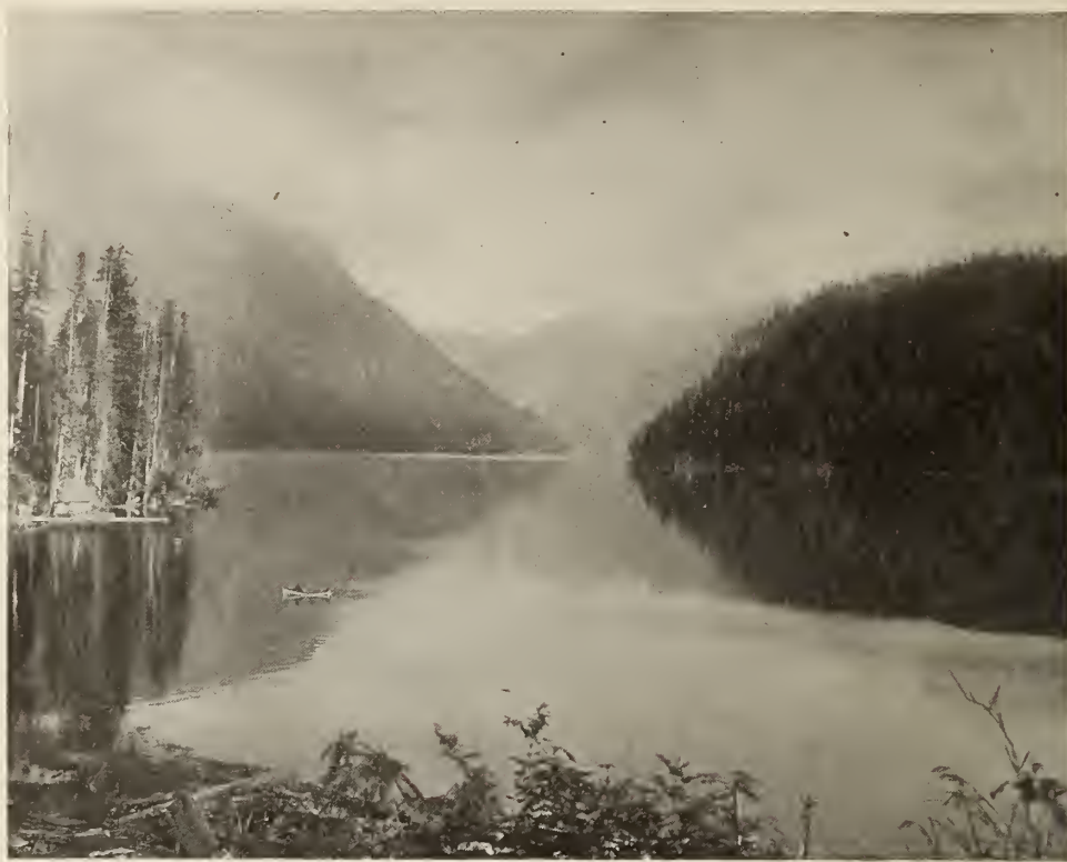
Coquitlam Lake with dam in background, Coquitlam-Buntzer Development
