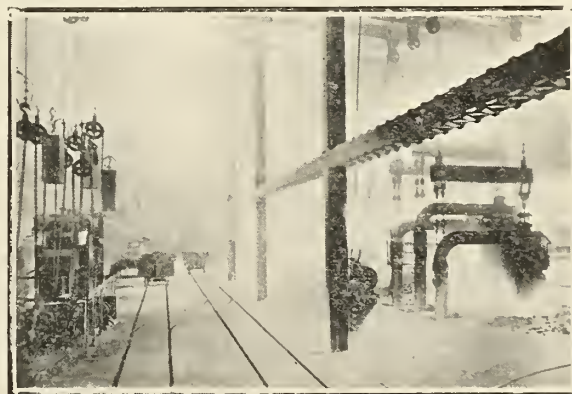
One of the carbide furnaces in American Cyanamid Co.'s Plant
