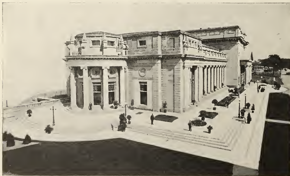
Power House, Electrical Development Company, Niagara Falls, Ont.
