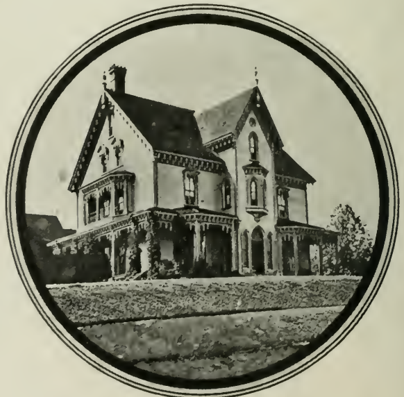
ALEXANDER GIBSON'S RESIDENCE
