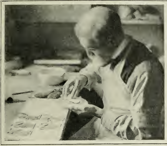
(Photo: Clarke & Hyde.) THE METHOD OF LAYING FIGURES ON CLAY SLABS. THIS WORKER HAS BEEN 53 YEARS WITH WEDGWOOD
