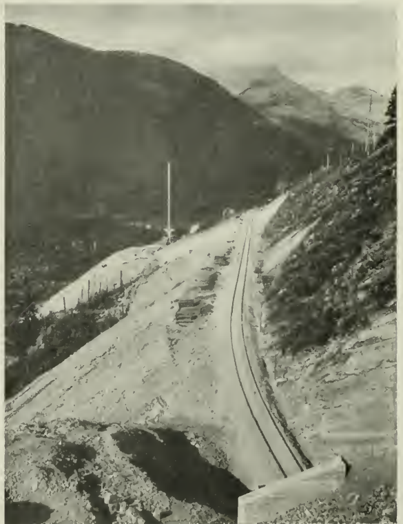
NEW SPIRAL TUNNEL ON THE C.P.R. NEAR FIELD, B.C. ARROW INDICATES THE ENTRANCE, WHILE THE EXIT IS IN THE IMMEDIATE FOREGROUND
