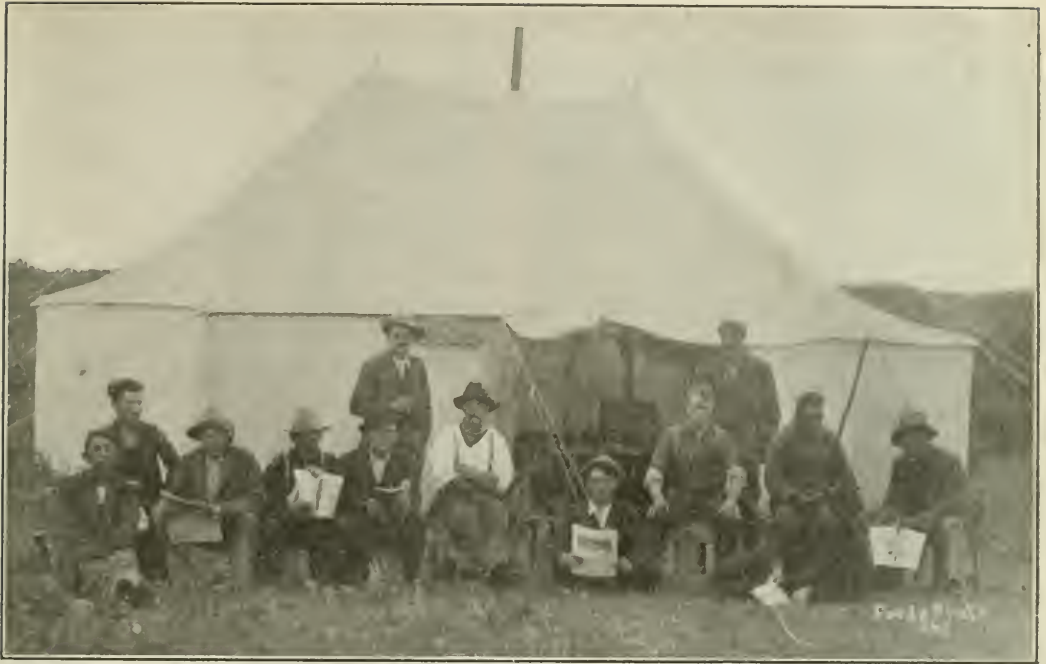
Camp Reading Tent, G.T.P. Construction, Touchwood Hills, Sask.
