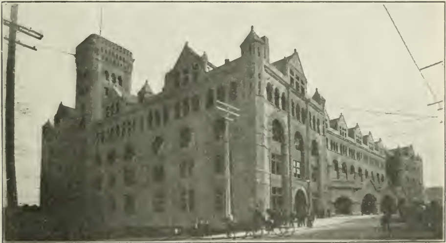
Windsor Street Station of C.P.R., Montreal.
