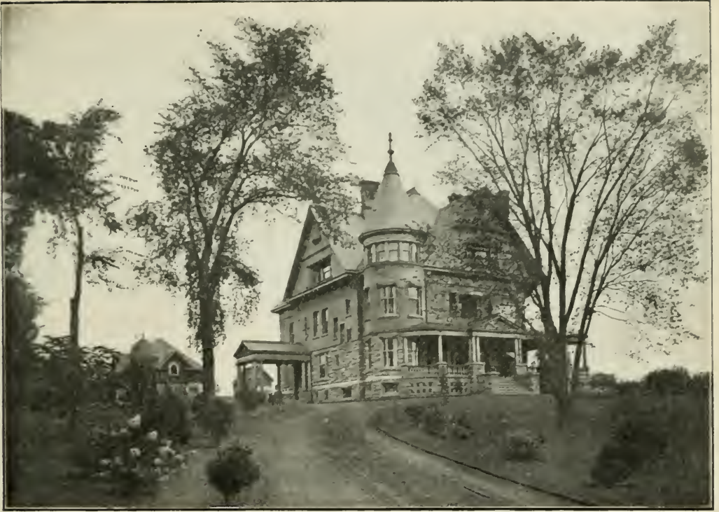
The Residence of Senator Frost, Smith's Falls, Ont.
