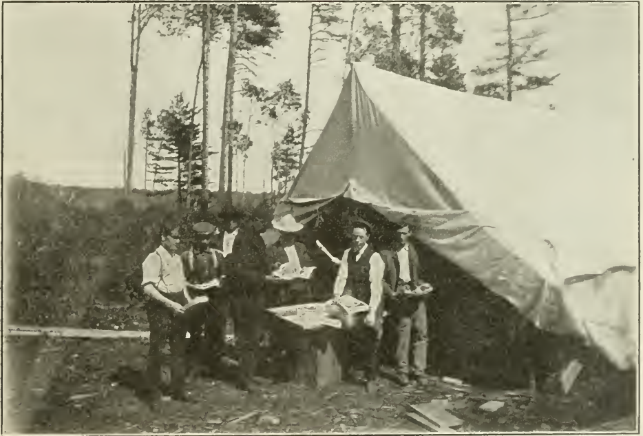
Reading Tent, T. & N.O. Railway Construction.
