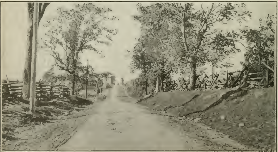
A Well Gravelled and Thoroughly Drained Road in Hastings County.
