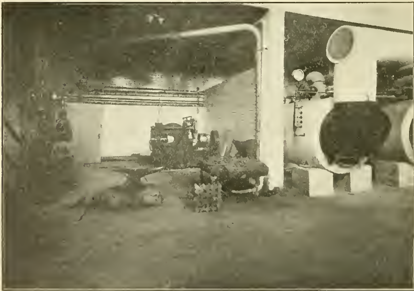
Fig. 10—Boiler House and Smith's Shop.
