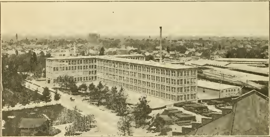
Example 4. Factory of German American Button Co., Rochester, N.Y. Building in Foreground is of Plain Monolithic Reinforced Concrete Without Brick Veneer or Trim of any Kind.
