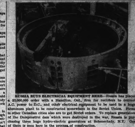
RUSSIA BUYS ELECTRICAL EQUIPMENT HERE—Russia has placed a $3,000,000 order with a Hamilton, Ont., firm for rectifiers to convert A.C. power to D.C., and other electrical equipment to be used in a huge aluminum plant to be constructed somewhere in the Soviet Union. Firms in other Canadian cities also are to get Soviet orders. To replace generators of the Dneprostrai dam which were destroyed in the war, Russia is purchasing three huge hydro-electric generators at Schenectady, N.Y. One of them is seen here in the process of construction.
