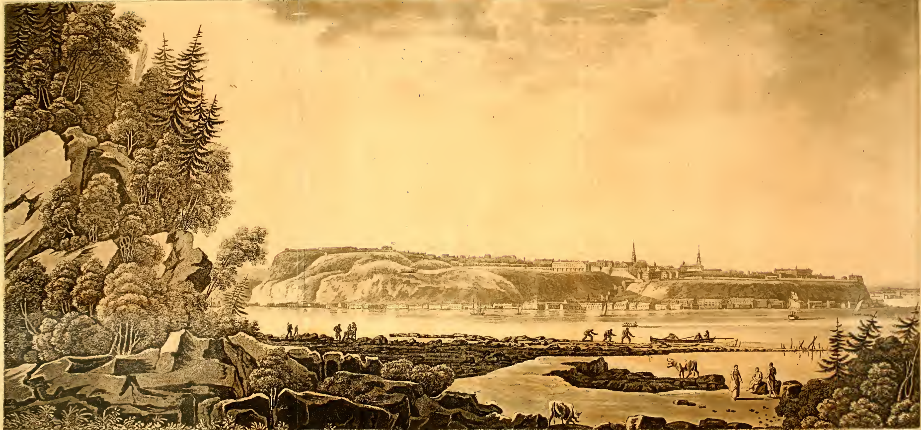
View of Quebec as taken from Point Lévis
