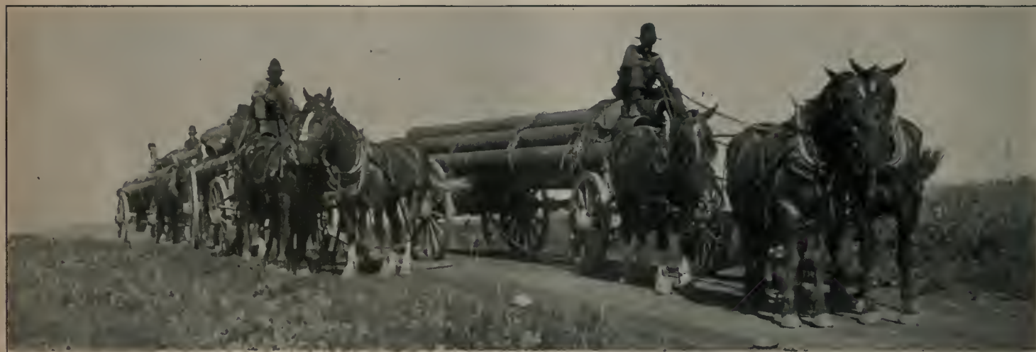
THE BIG TEAMS THAT HAUL CASING TO THE WELLS
