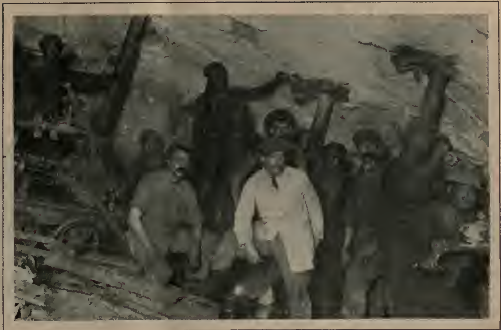
Shaft sinking on the Village Deep Gold Mine
