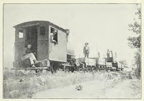
A CONVICT-MANAGED RAILWAY IN OPERATION The Prison Farm uses a railway system extending over two and a half miles for stone transportation, on which prisoners act engineer, fireman and brakeman
