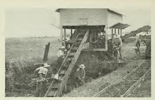
THE END ELEVATION OF A PEAT MACHINE, SHOWING THE ELEVATOR WHICH (ARRIES THE PEAT OUT OF THE TRENCH, MEN AT WORK DIGGING THE PEAT AND THE TRACK ON WHICH THE CARS TRAVEL WHICH HAUL THE PEAT AWAY
