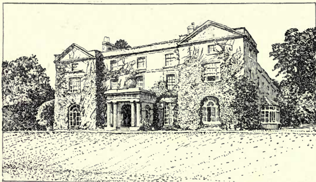
THE RESIDENCE KNOWN AS HEMBURY FORT.
