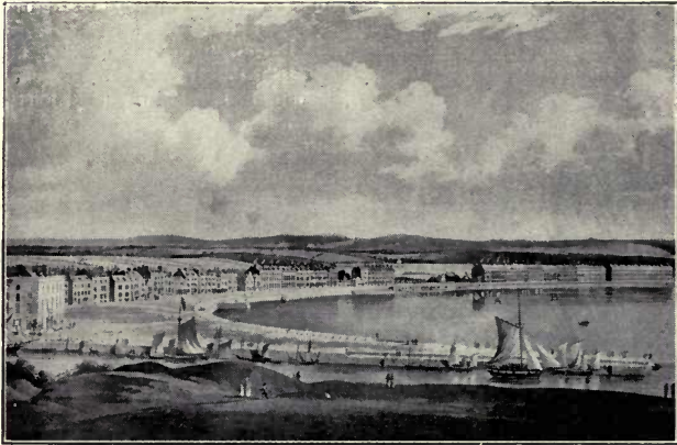
VIEW OF WEYMOUTH, LOOKING WEST. A B
