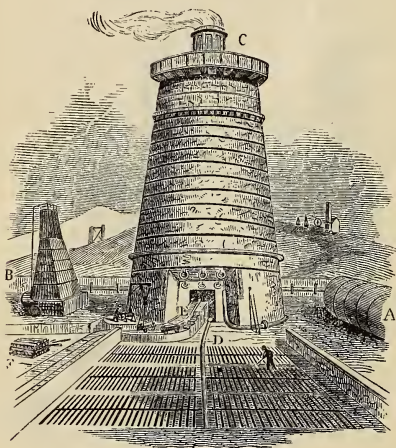
Outward view of Blast-furnace, showing (at D) the molten iron running off into the moulds to form pig-iron.
