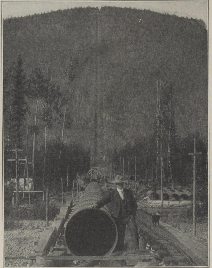
*A Water Flume for Gold Mining in the Yukon*
