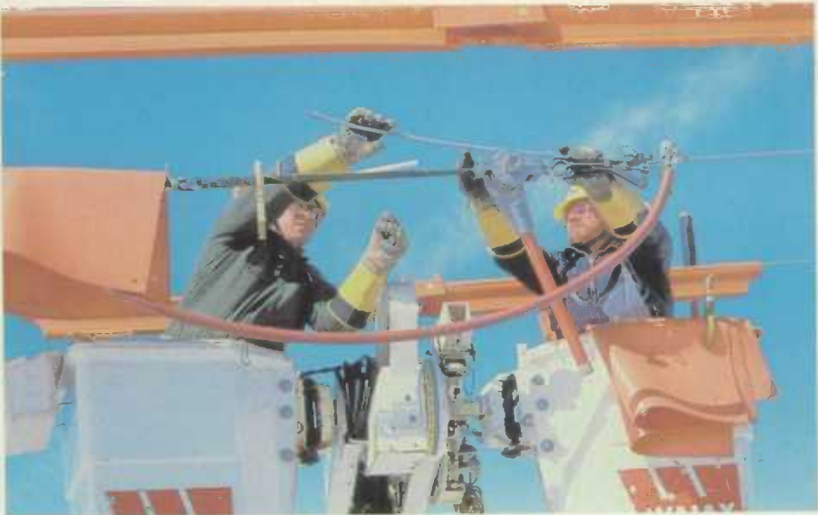
Hydro line repairmen at Mactaquac, NB.
