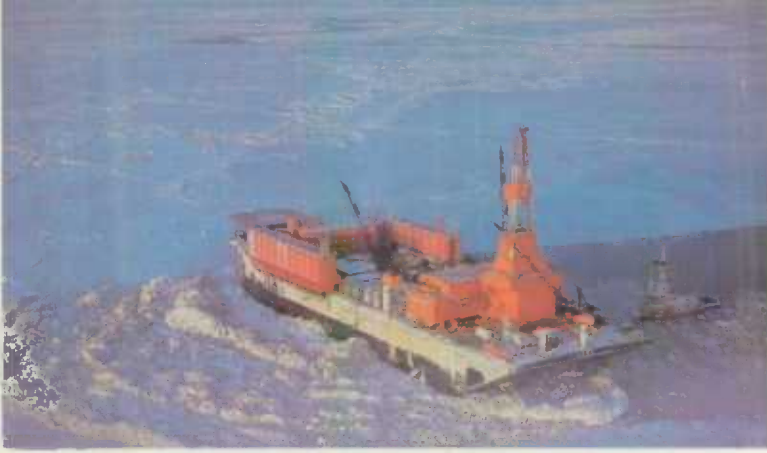
Dome's drilling island system, the SSDC (single steel drilling caisson) sets on an underwater sand foundation and can operate outside the stable landfast ice area, in the unpredictable shear ice zone.
