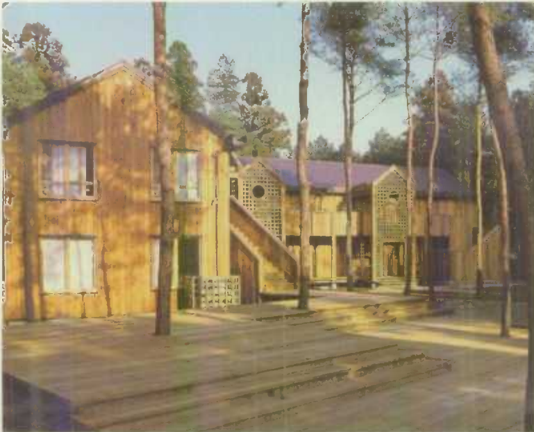
Houses in Tskuba, Japan, built with lumber from Canada.
