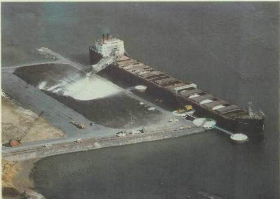
Unloading a cargo of salt at the bulk materials wharf, recently constructed at Morrisburg, Ont.
