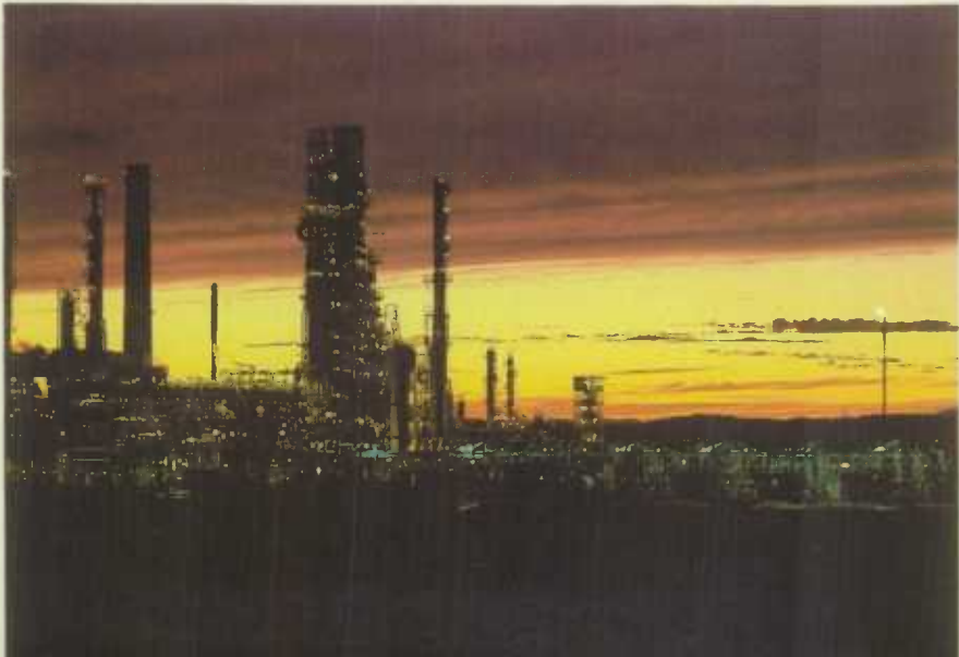
Oil refinery near Quebec City, Que.
