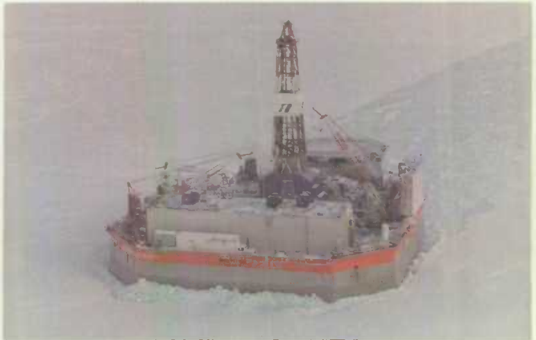
Gulf's MOLIKPAQ, an extension of the caisson-retained island concept, is the first single-piece deep caisson vessel designed and constructed for bottom-founded year-round drilling operations in Arctic waters.
