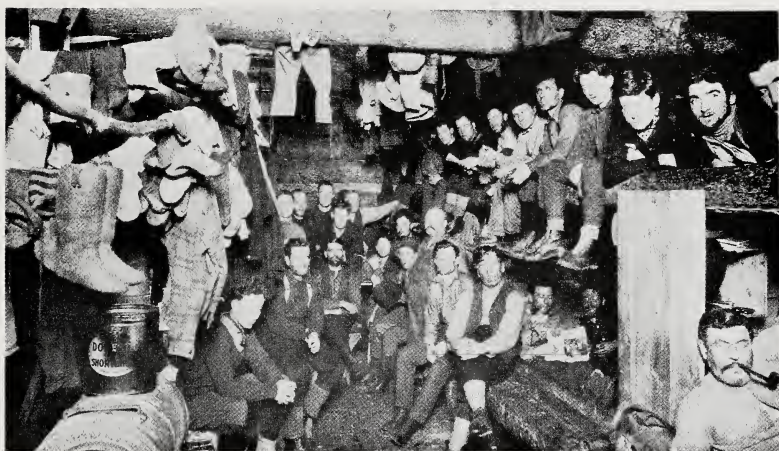
Interior of workers' bunkhouse.
