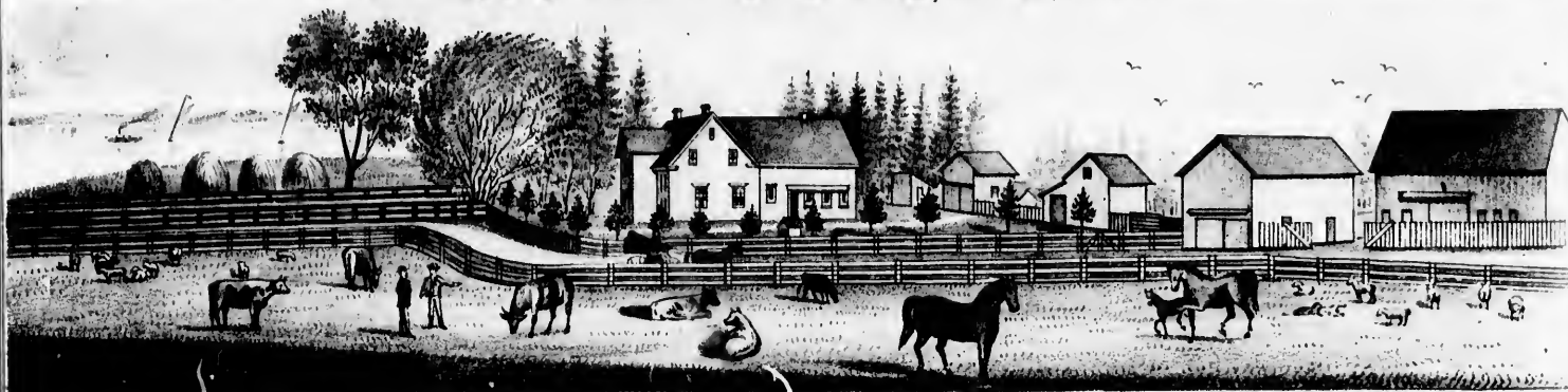
"POINT PLEASANT" FARM RES. OF D. H. Mc DONALD ESQ. NORTH BEDEQUE, LOT 25, P. E. I.
