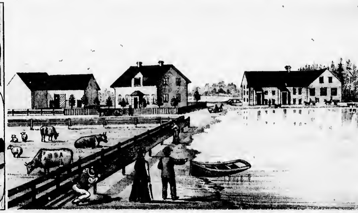
RES. & MILL PROPERTY OF EDW. J. WRIGHT, NEW ANNAN MILLS, LOT 19, P. E. I.
