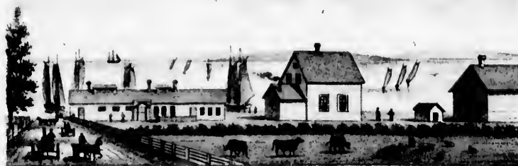
I B. HAMBLÉN & CO LOBSTER CANNING FACTORY & RESIDENCE, WOOD ISLANDS, LOT 62, PEI
