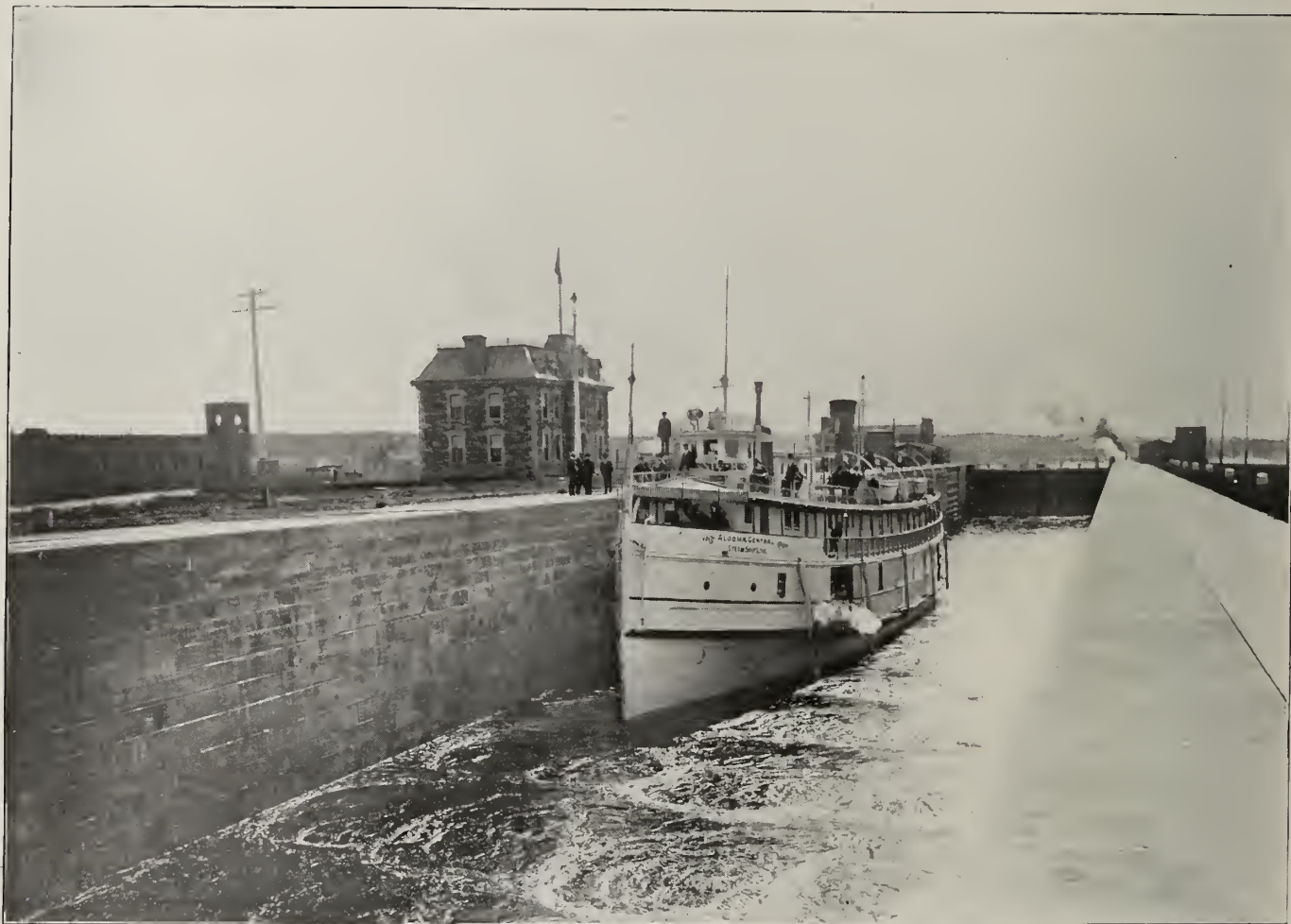
ANOTHER VIEW OF THE CANADIAN LOCK.
