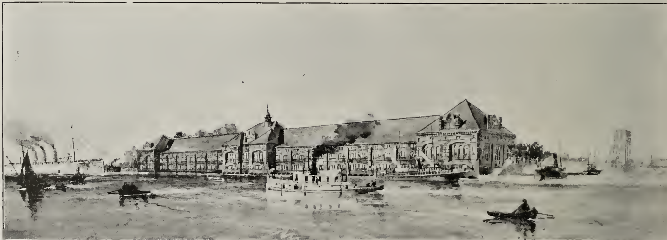
POWER HOUSE OF THE MICHIGAN LAKE SUPERIOR POWER COMPANY
