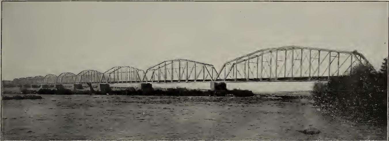
INTERNATIONAL BRIDGE ACROSS THE ST. MARV'S RIVER AT SAULT STE. MARIE—OWNED BY THE CANADIAN PACIFIC RAILWAY.
