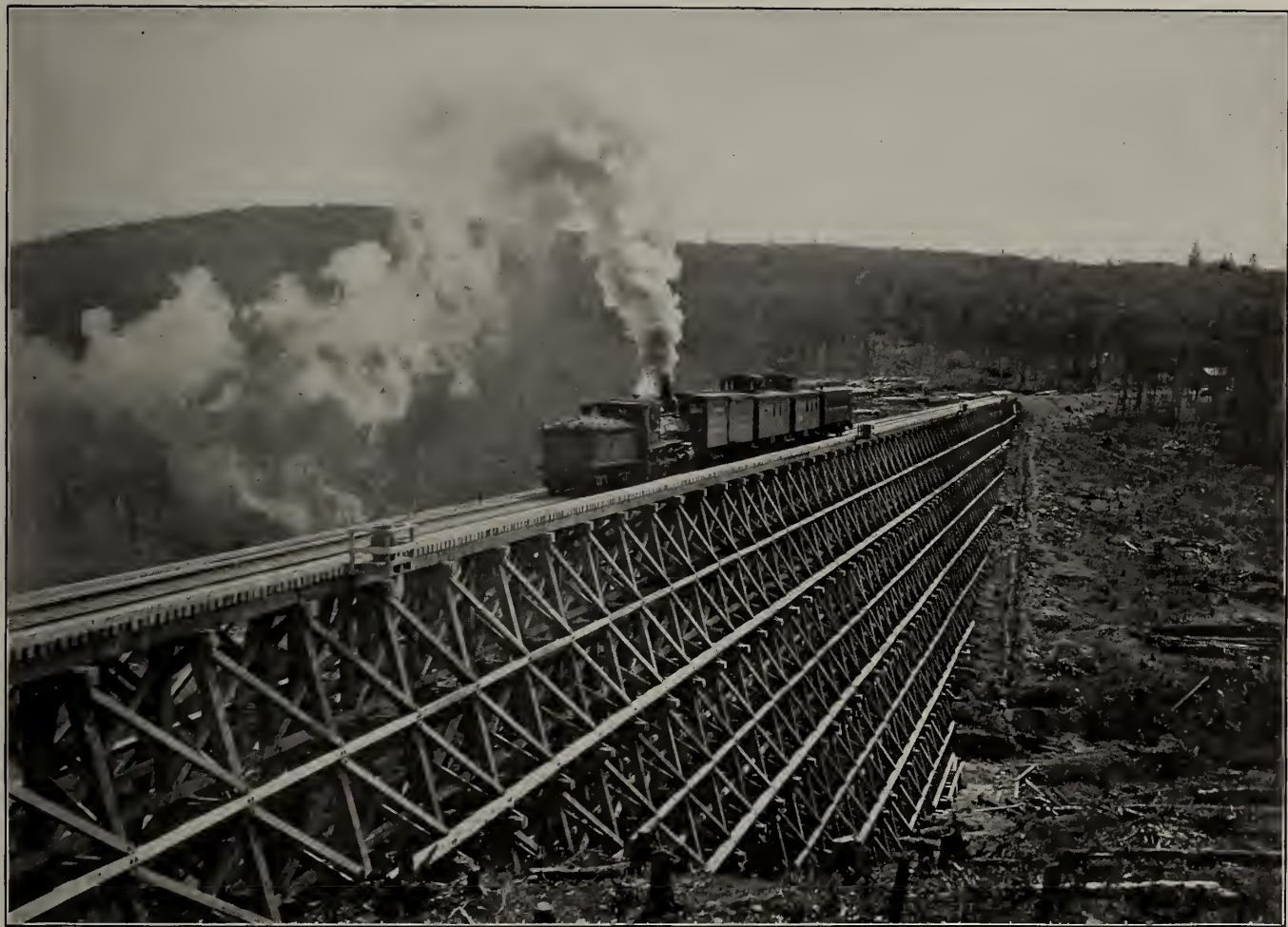
BELLEVUE TRESTLE—ONE OF THE LARGEST IN CANADA.
