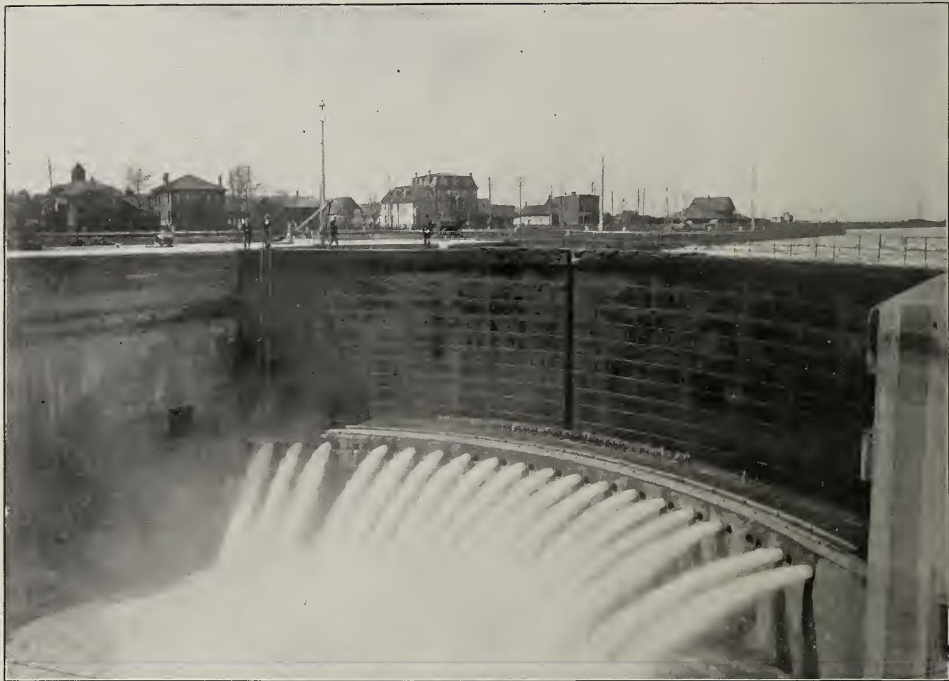
FILLING THE UNDER CHANNELS OF POE LOCK PREPARATORY TO OPENING FOR NAVIGATION.
