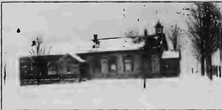
HALF OF THIS SCHOOL NOW UNUSED. NO IMPROVEMENTS IN MANY YEARS.
