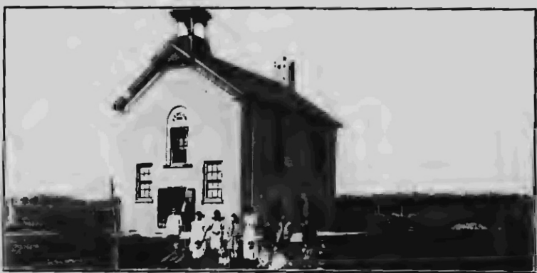
ONE OF THE BETTER TYPE OF SCHOOL BUILDINGS.
