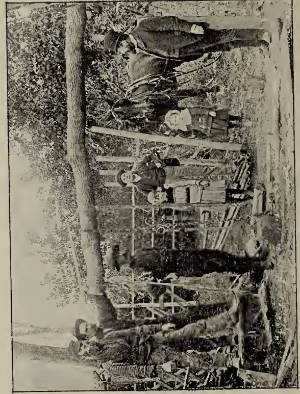
FIRST SYSTEM OF DRILLING (SPRING POLE).
