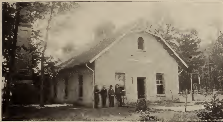
WATERWORKS ENGINEER'S RESIDENCE, LAKE HURON.
