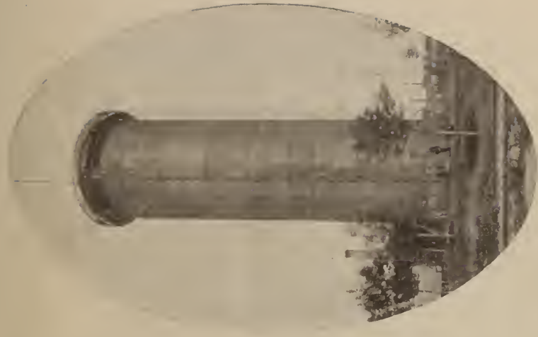
WATERWORKS STAND PIPE.
