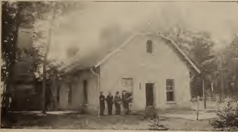
WATERWORKS PUMPING STATION, LAKE HURON,
