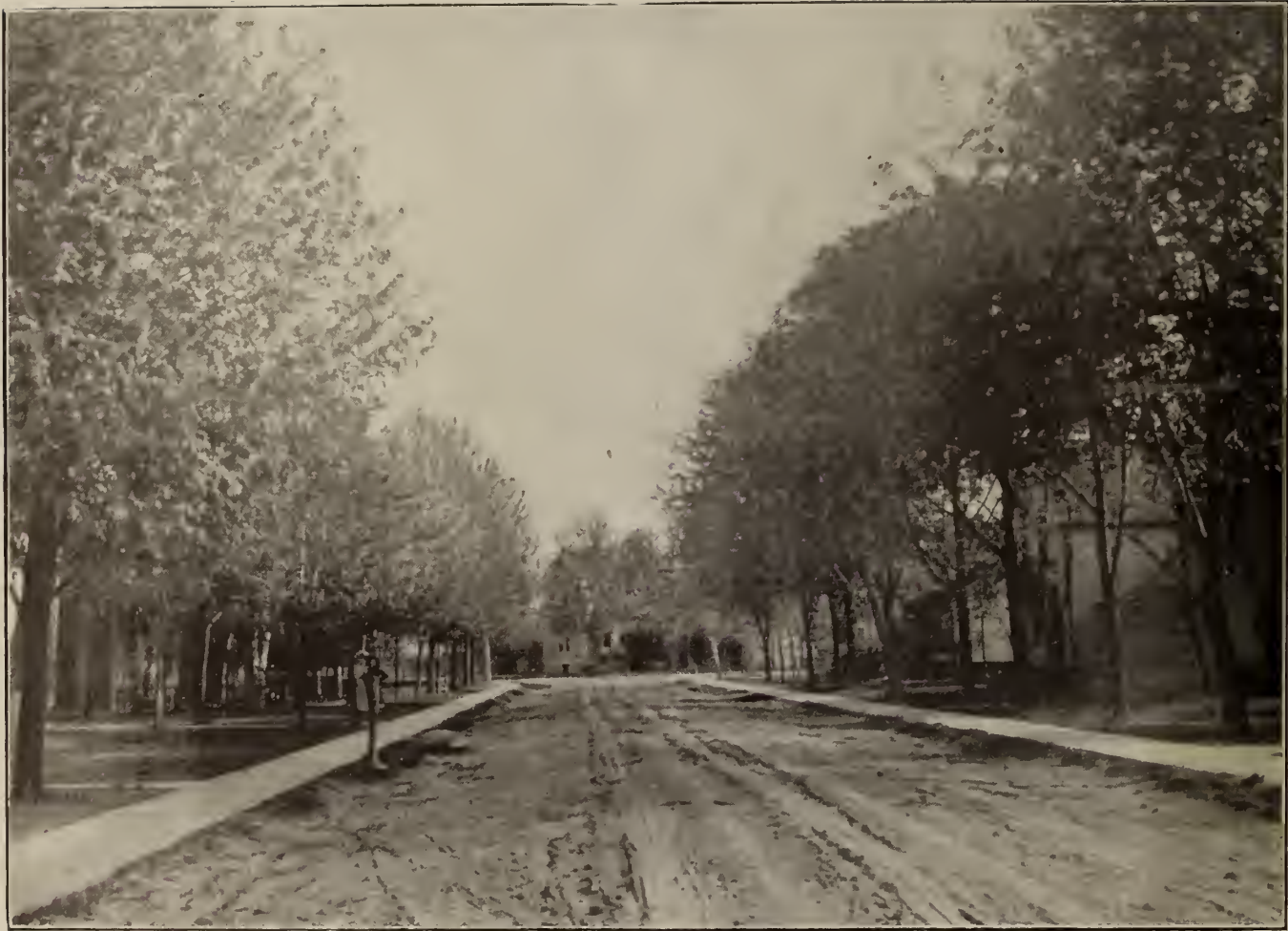
KING STREET (LOOKING SOUTH)
