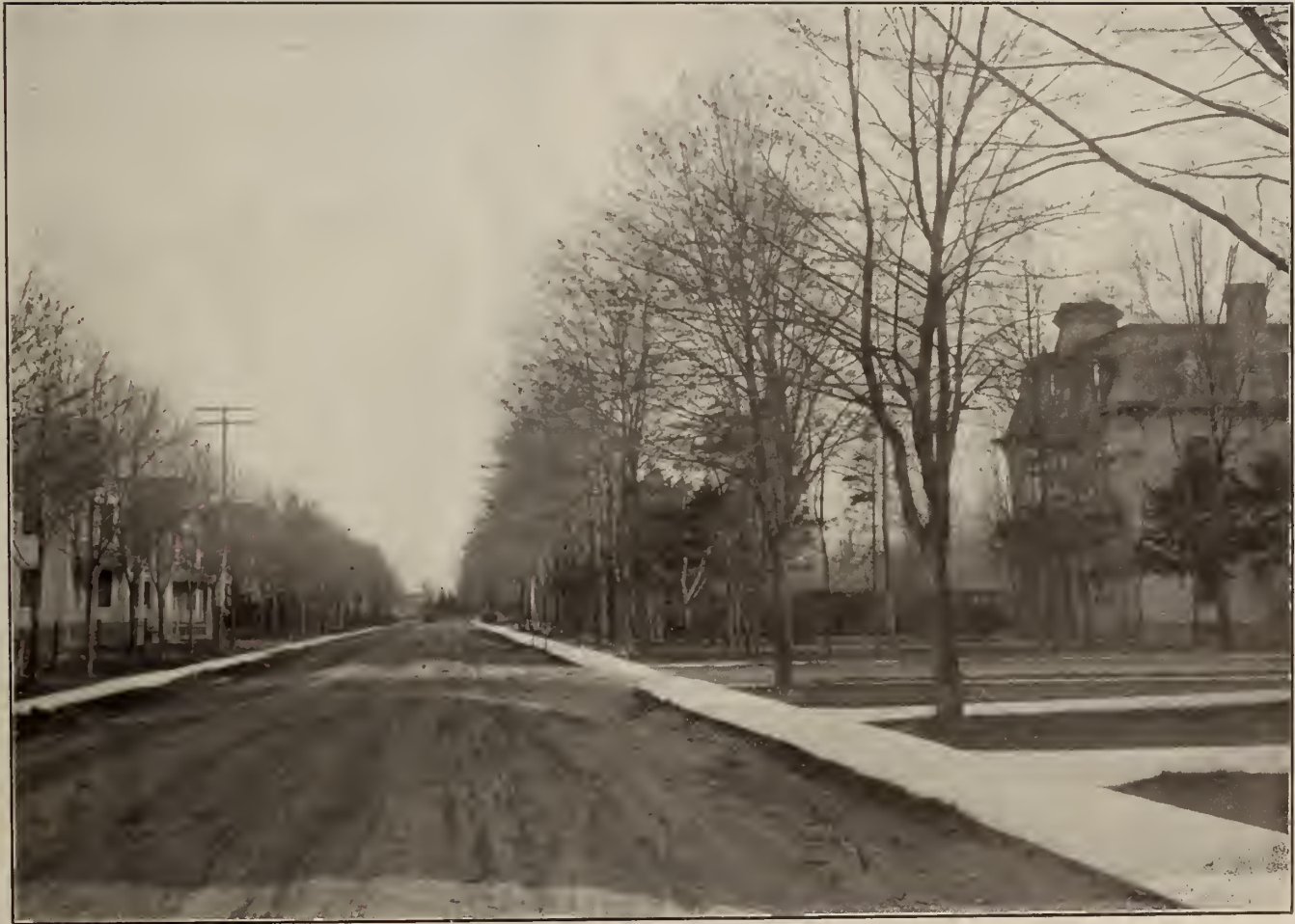
KING STREET (LOOKING SOUTH).
